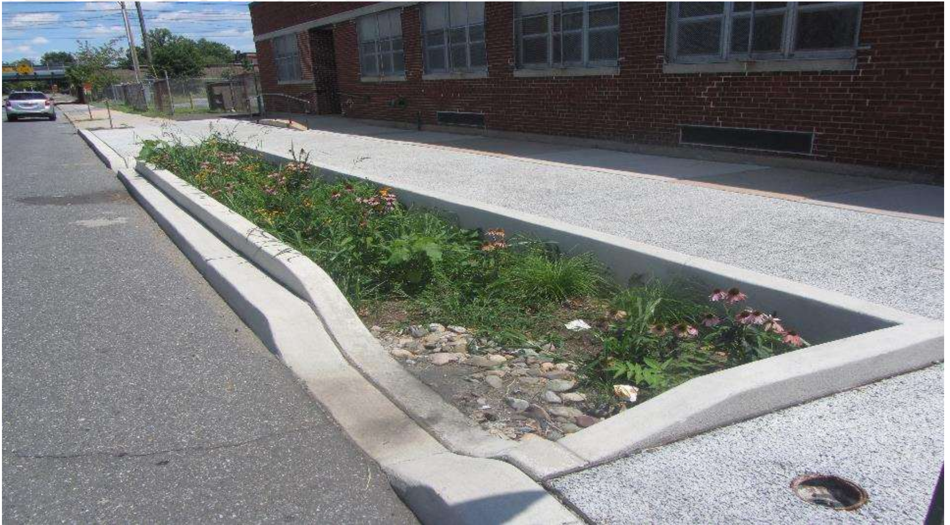
Stormwater Planter at the Brimm School in Camden, NJ Vegetative System
