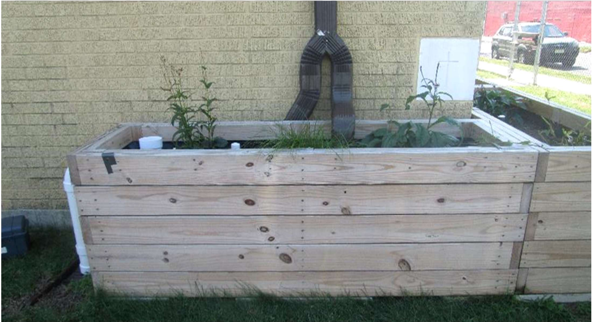
Downspout Planter Boxes at Acelero Learning Center in Camden, NJ Harvesting System
