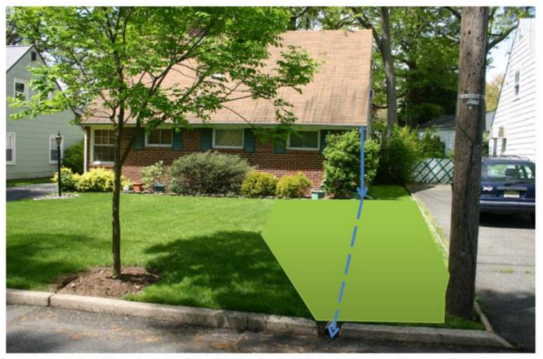
Downspout directly connected to street via metal pipe. Depending on slope/survey, downspout can be disconnected along the pipe or at the downspout. Catch basin installed into garden to connect overflow back into pipe.
