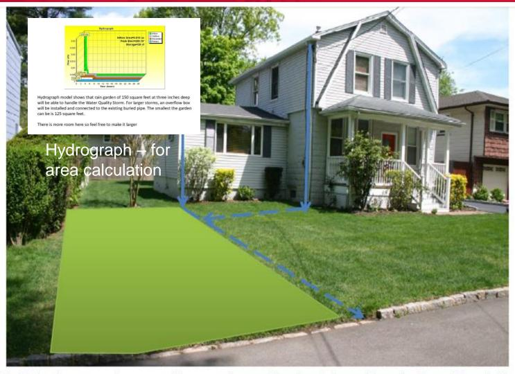
Multiple downspouts connect to one pipe out to street. I would prefer to not touch the pipe but rather build a garden along the curb cub (Minnesota Rain Garden) along with hardscaping/small retaining wall. But the pipe can be cut and a catch basin installed if
