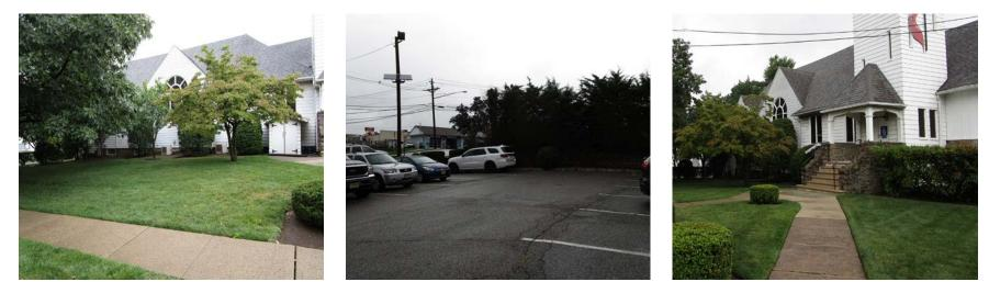
Parking spaces can be converted to porous pavement to capture and infiltrate stormwater runoff from the parking lot. Rain gardens can be installed in the turfgrass areas at the eastern side of the building to capture, treat, and infiltrate stormwater runoff from the roof if the downspouts are disconnected. A preliminary soil assessment suggests that the soils have suitable drainage characteristics for green infrastructure.
