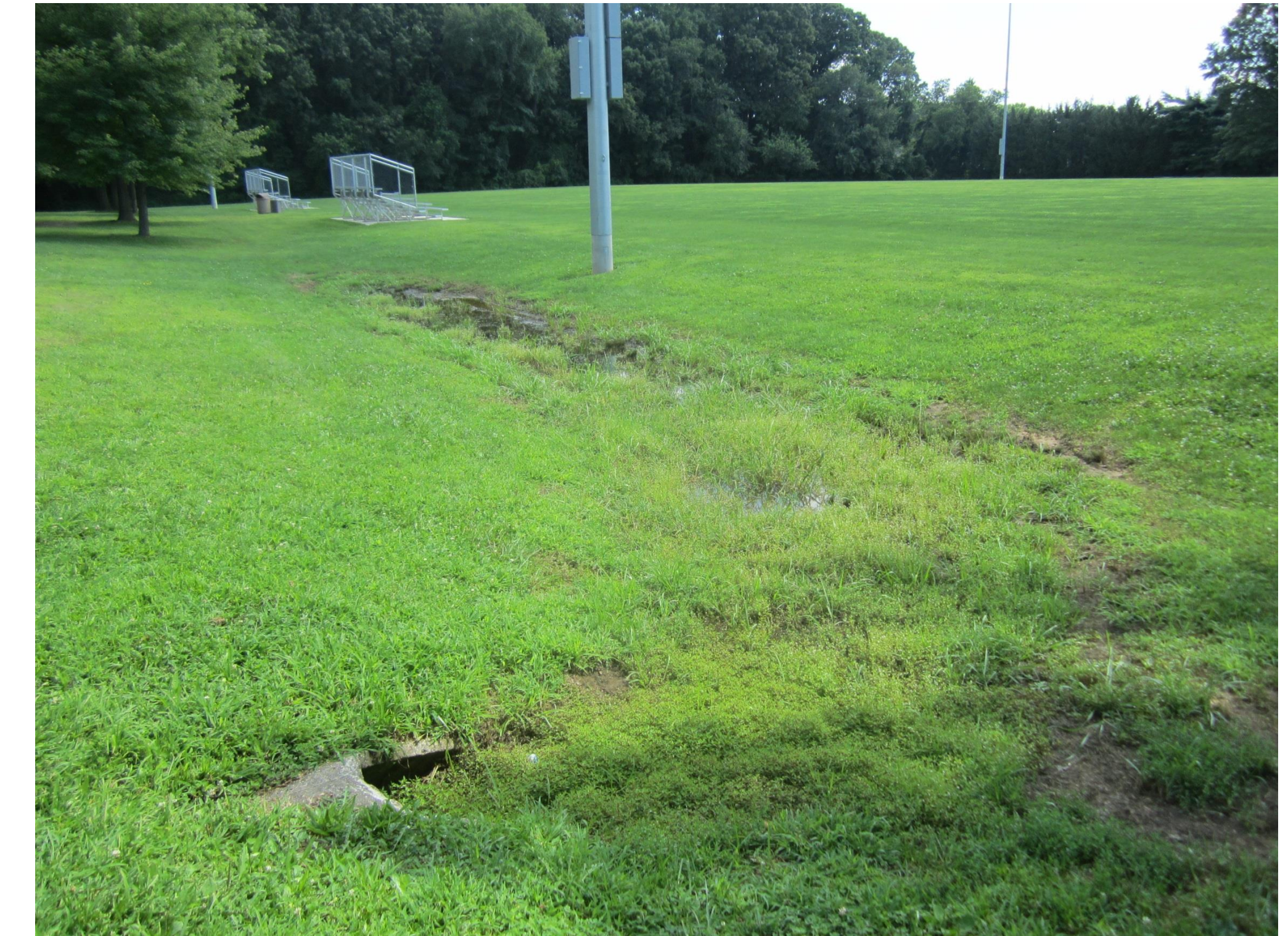
Basin #160 bottom looking north
