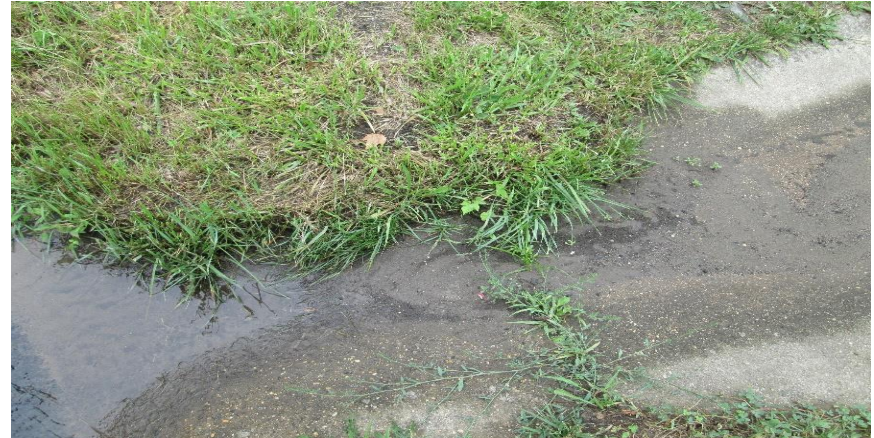
Low flow channel
