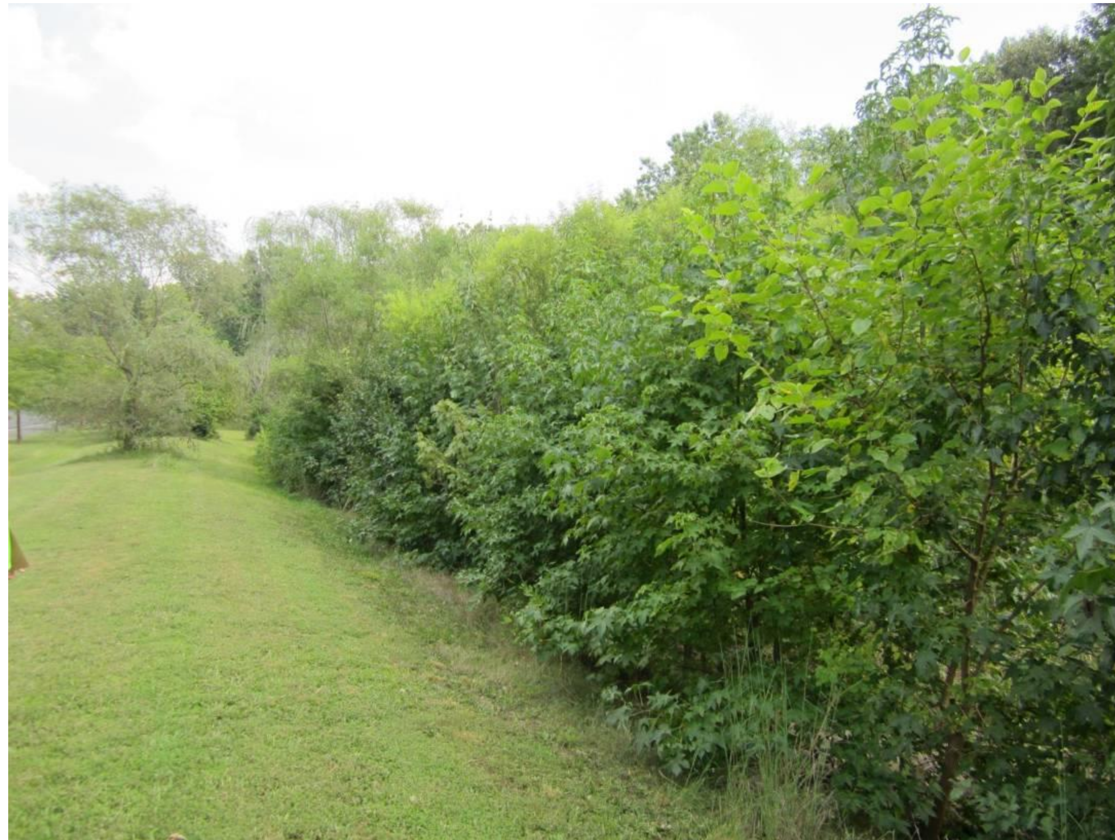
Basin bottom looking west
