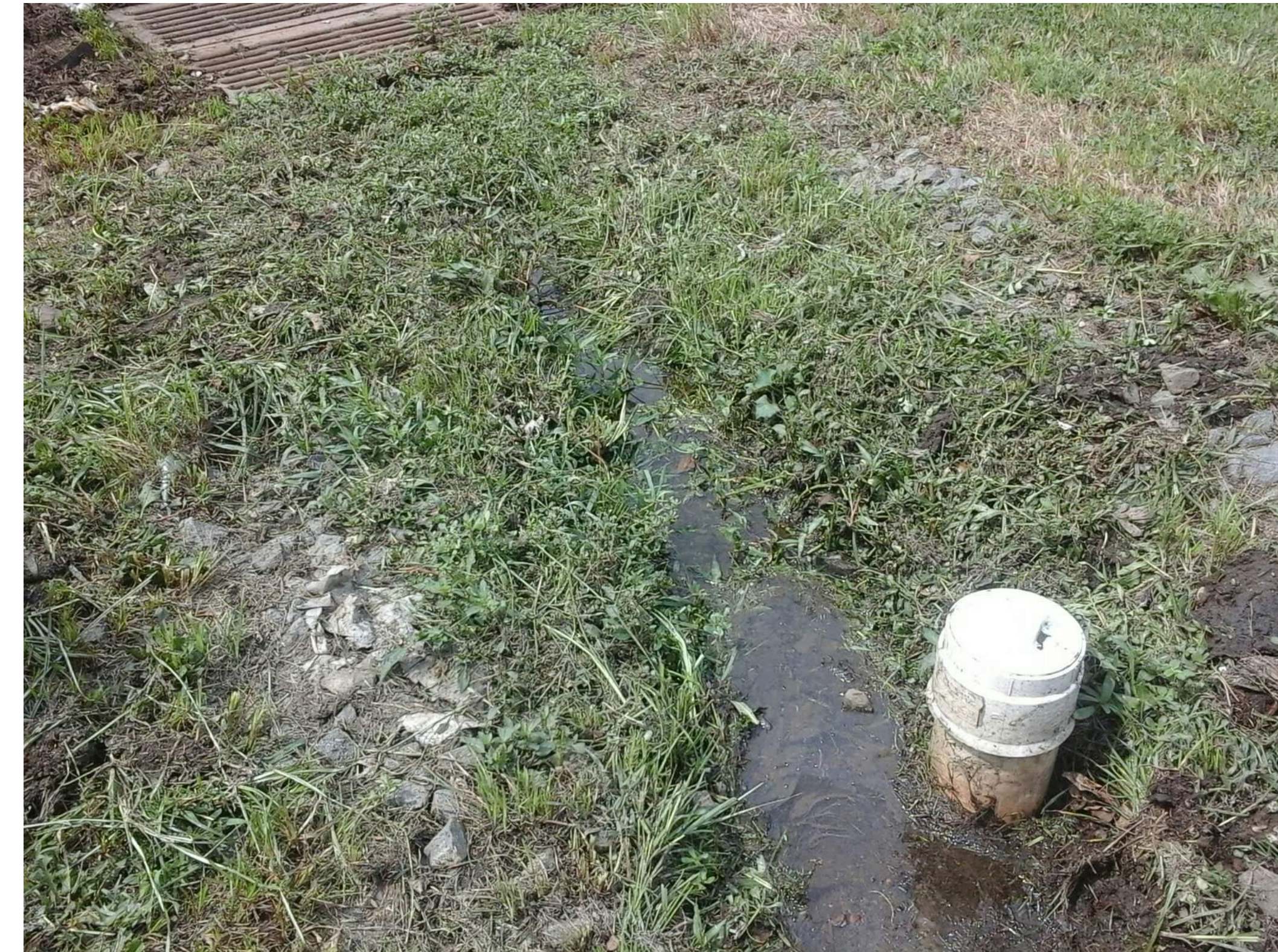
Clean out in low flow channel
