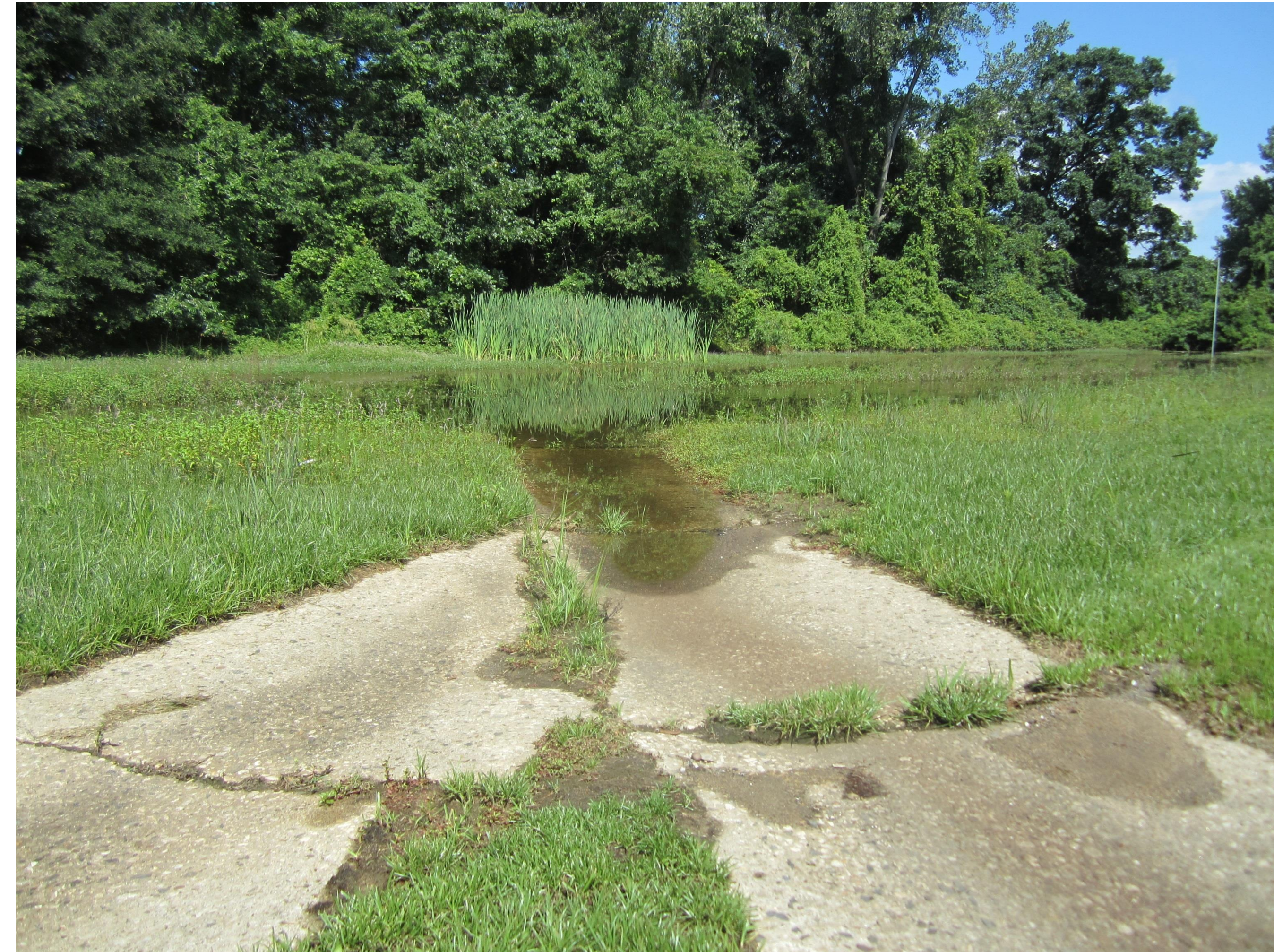
Basin bottom looking west
