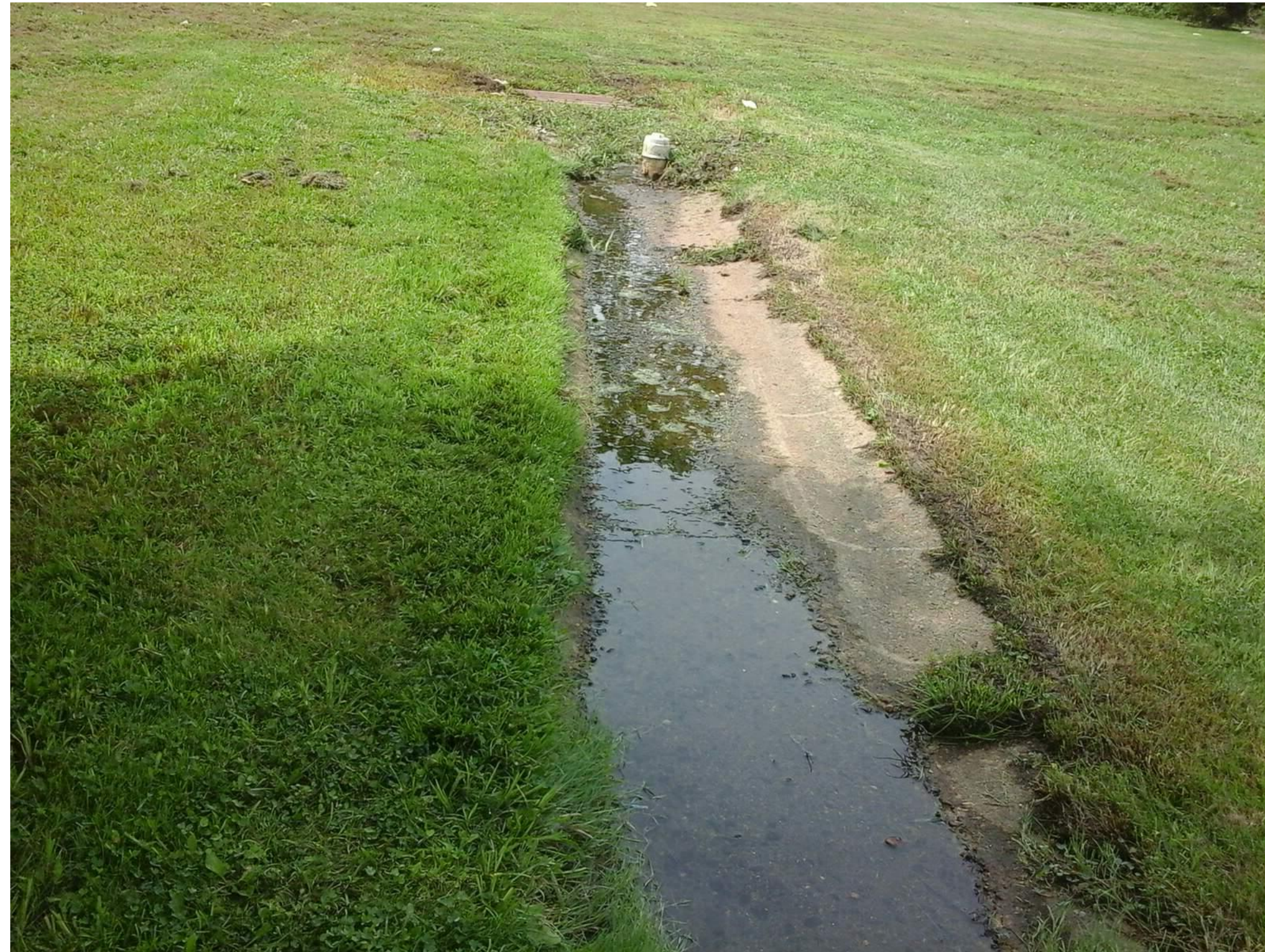
Low flow channel leading to catch basin
