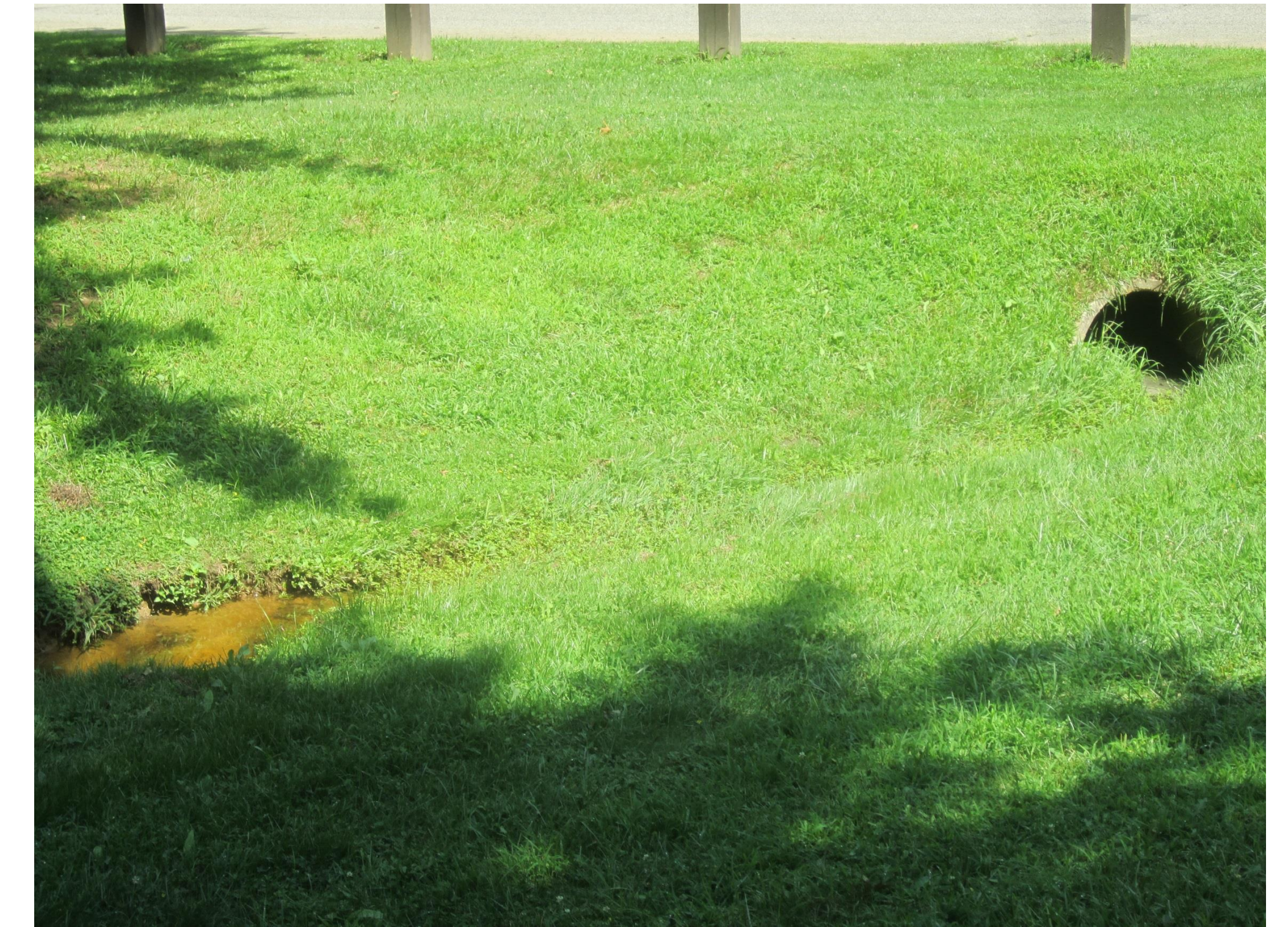
Outlet structure and gully
