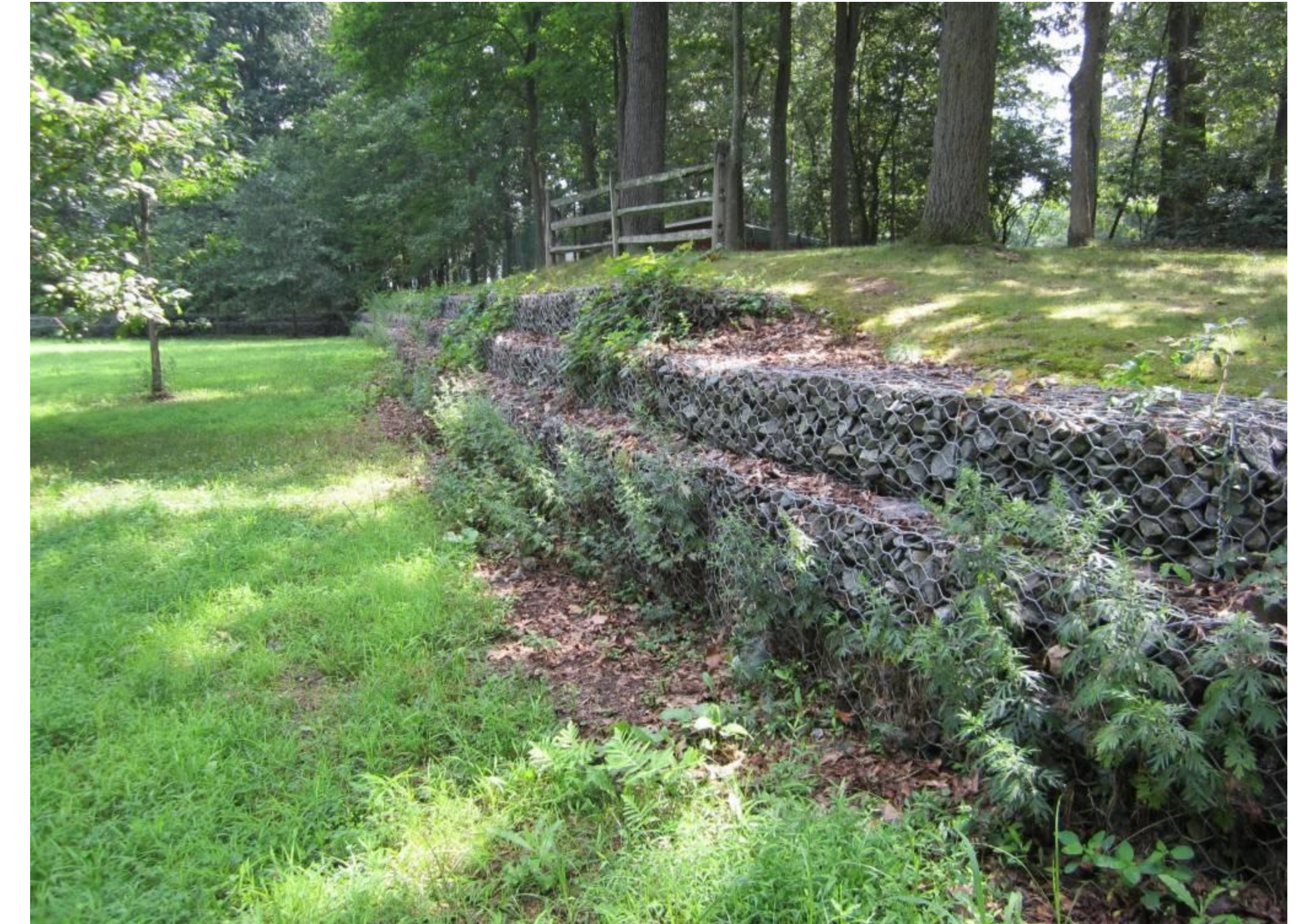
Gabion wall perimeter
