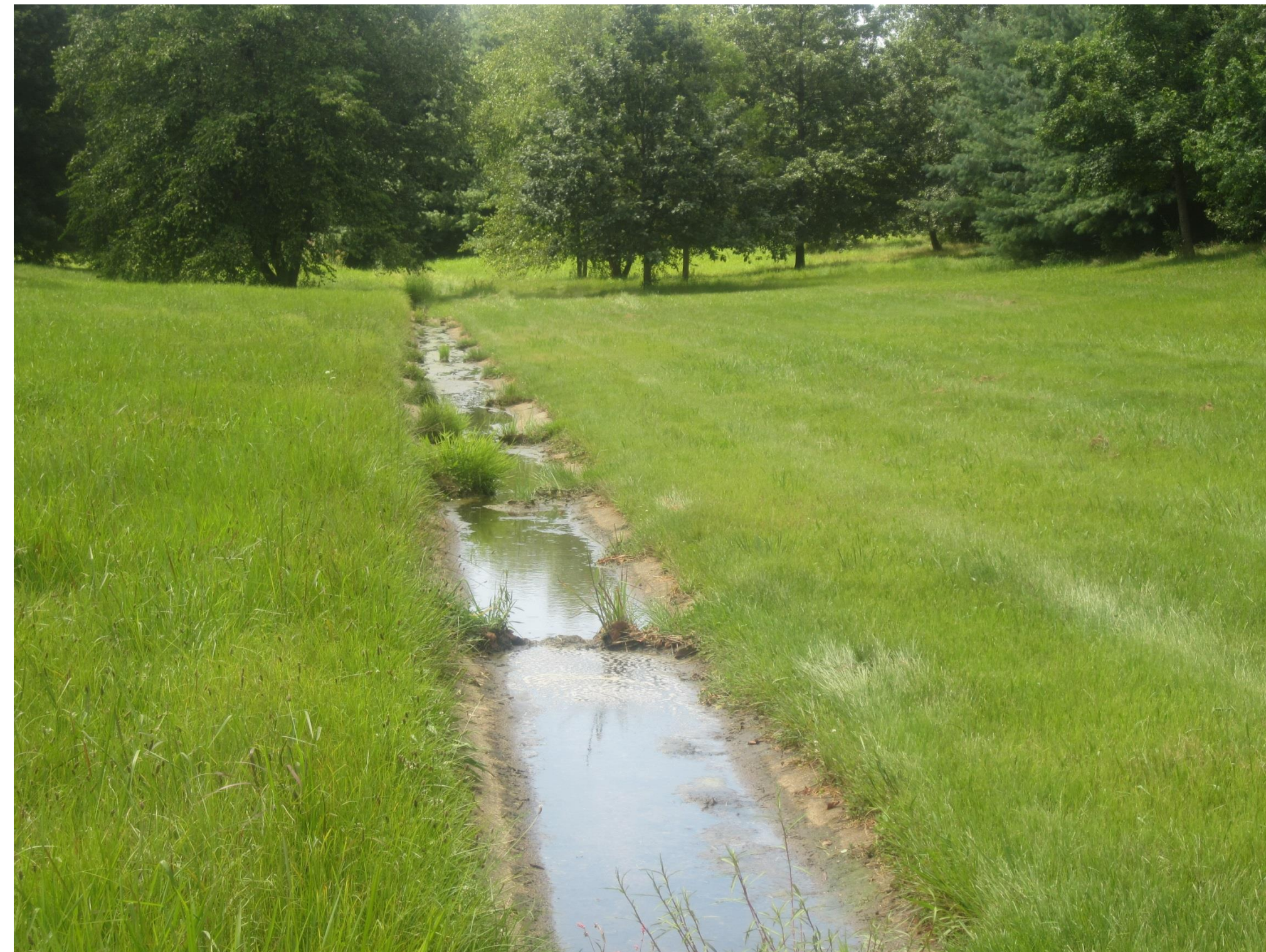
Basin bottom looking northwest
