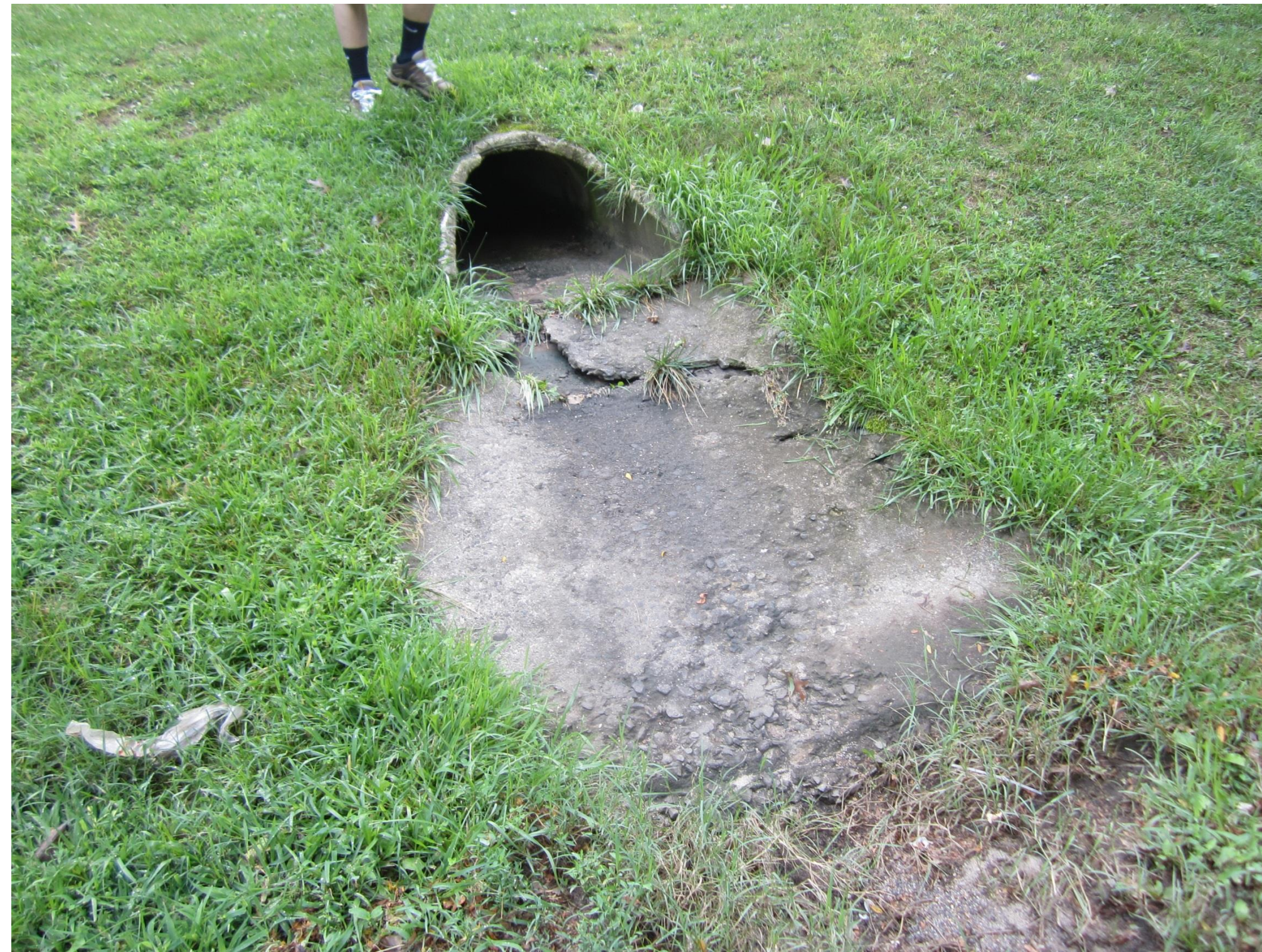
Northeastern inlet structure
