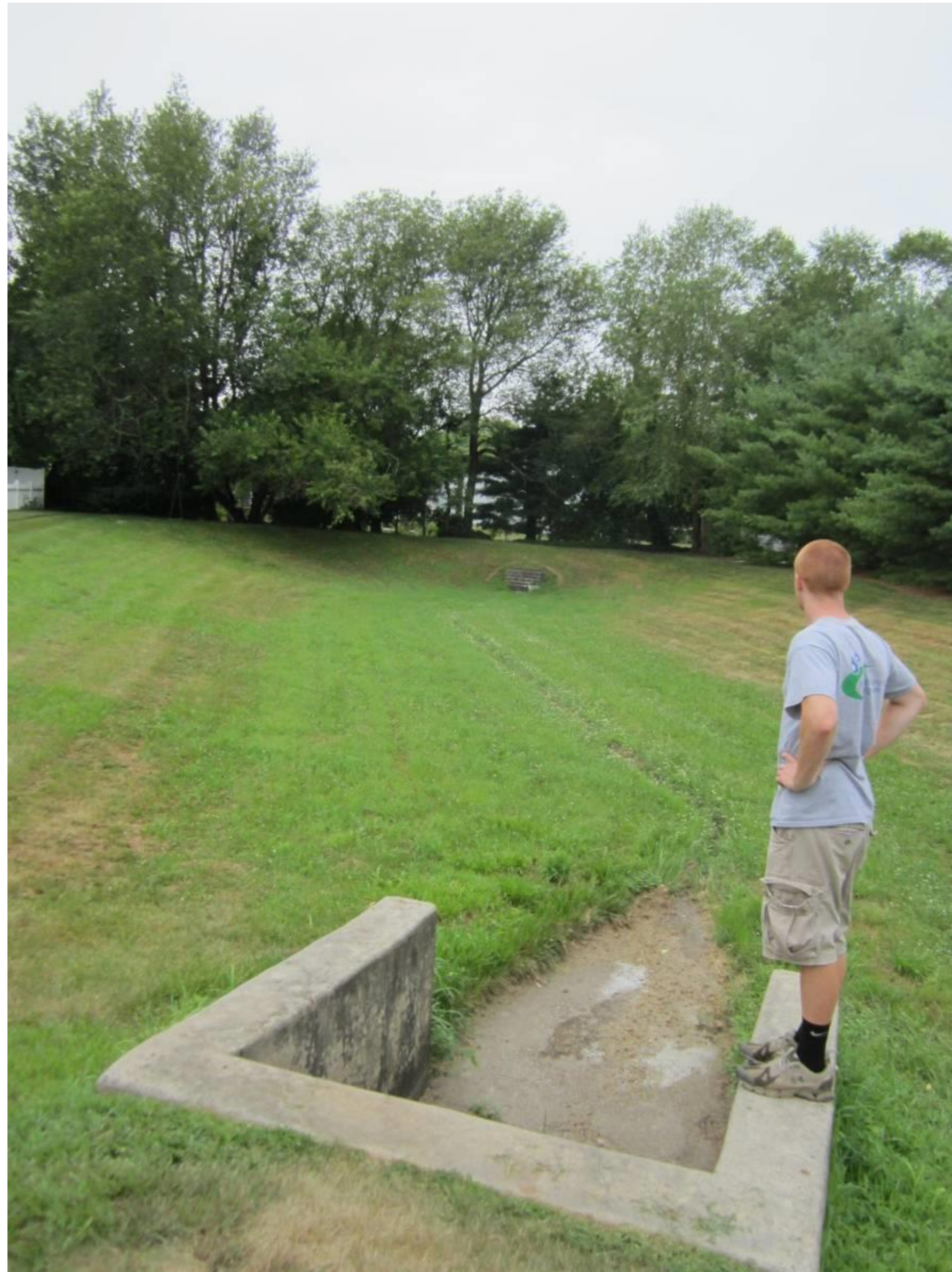
Basin bottom looking west
