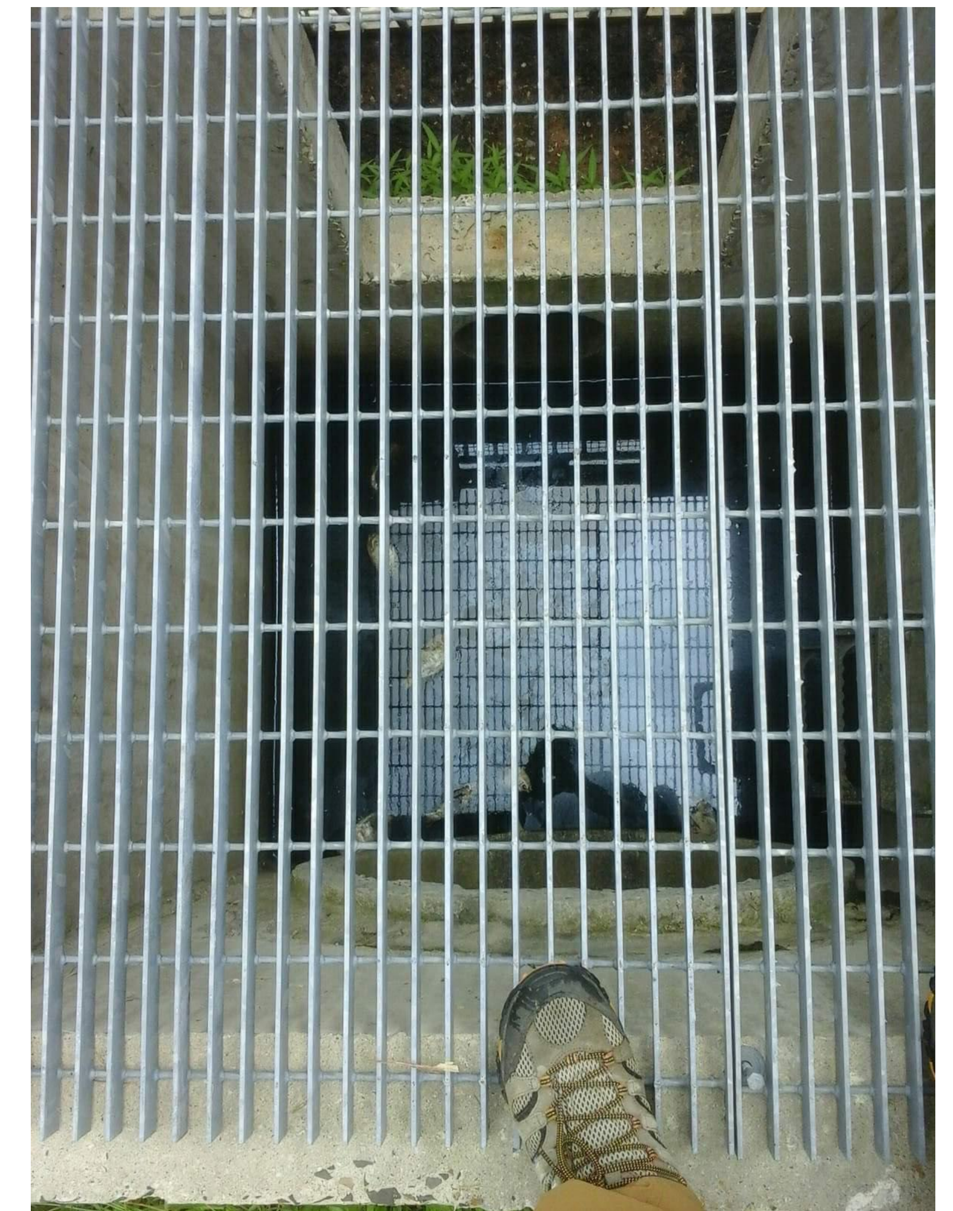
Fish in outlet structure
