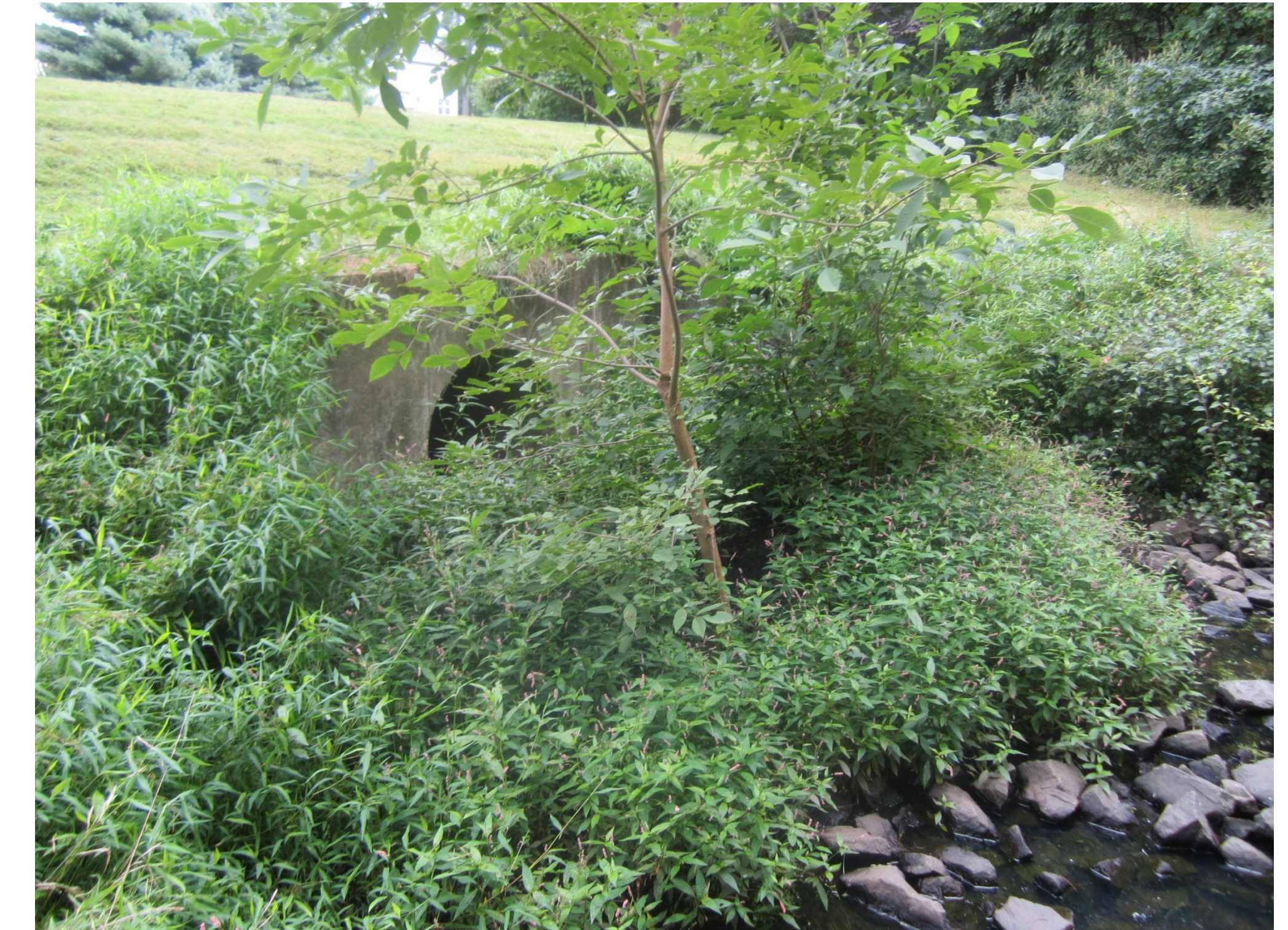
Basin discharge area
