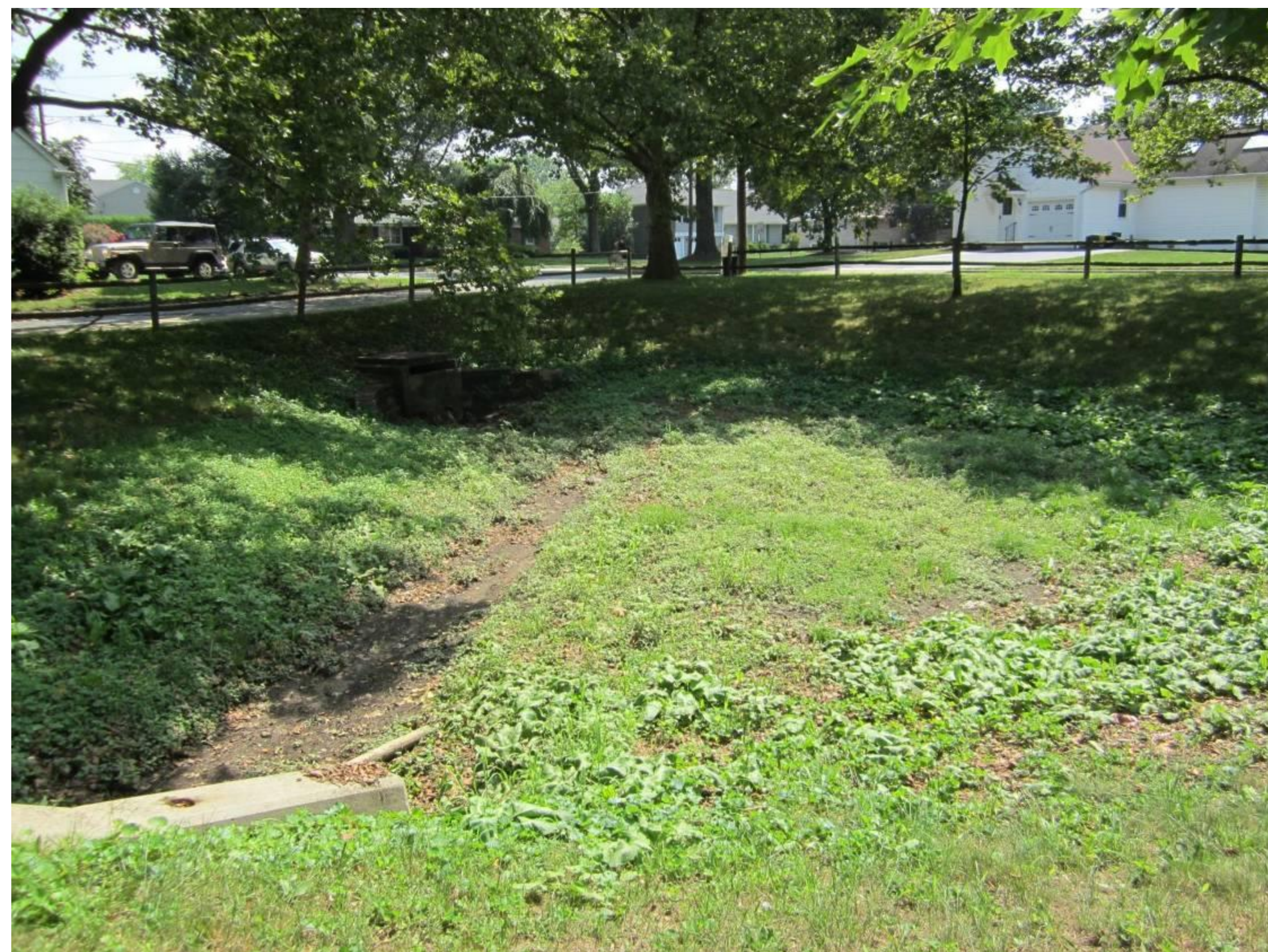
Basin bottom looking southeast
