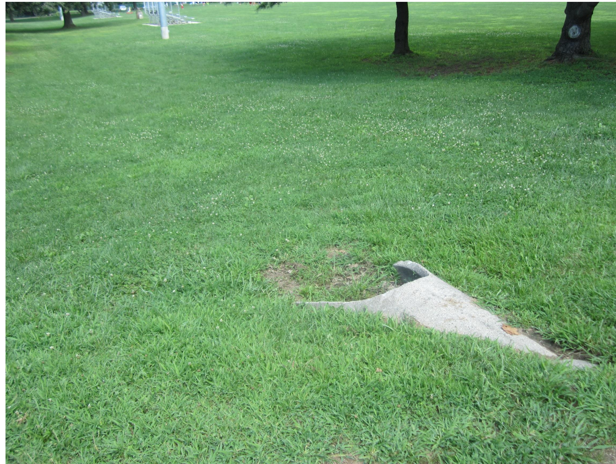
Basin #159 bottom looking west
