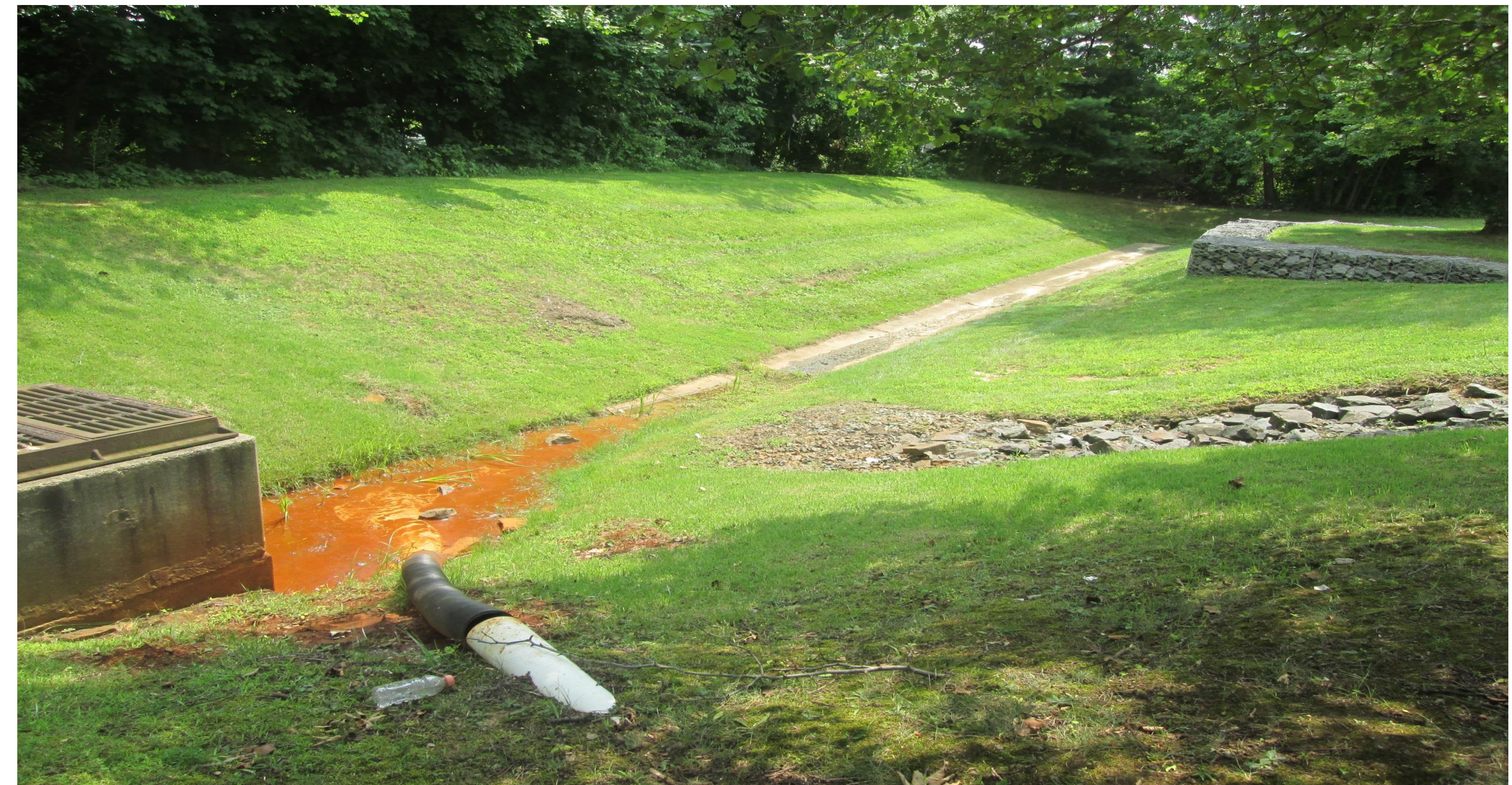
Overview of basin
