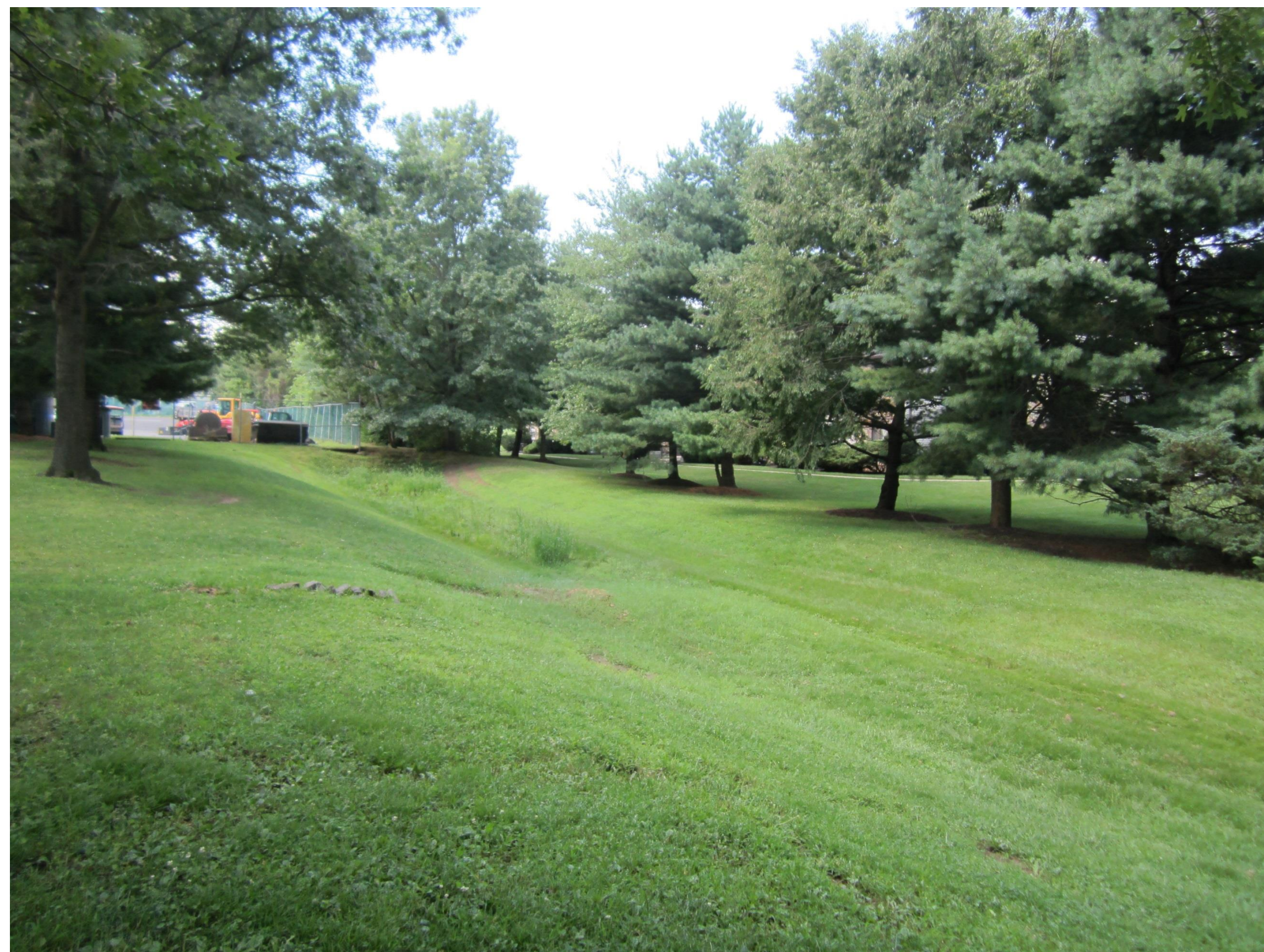
Basin bottom looking southwest
