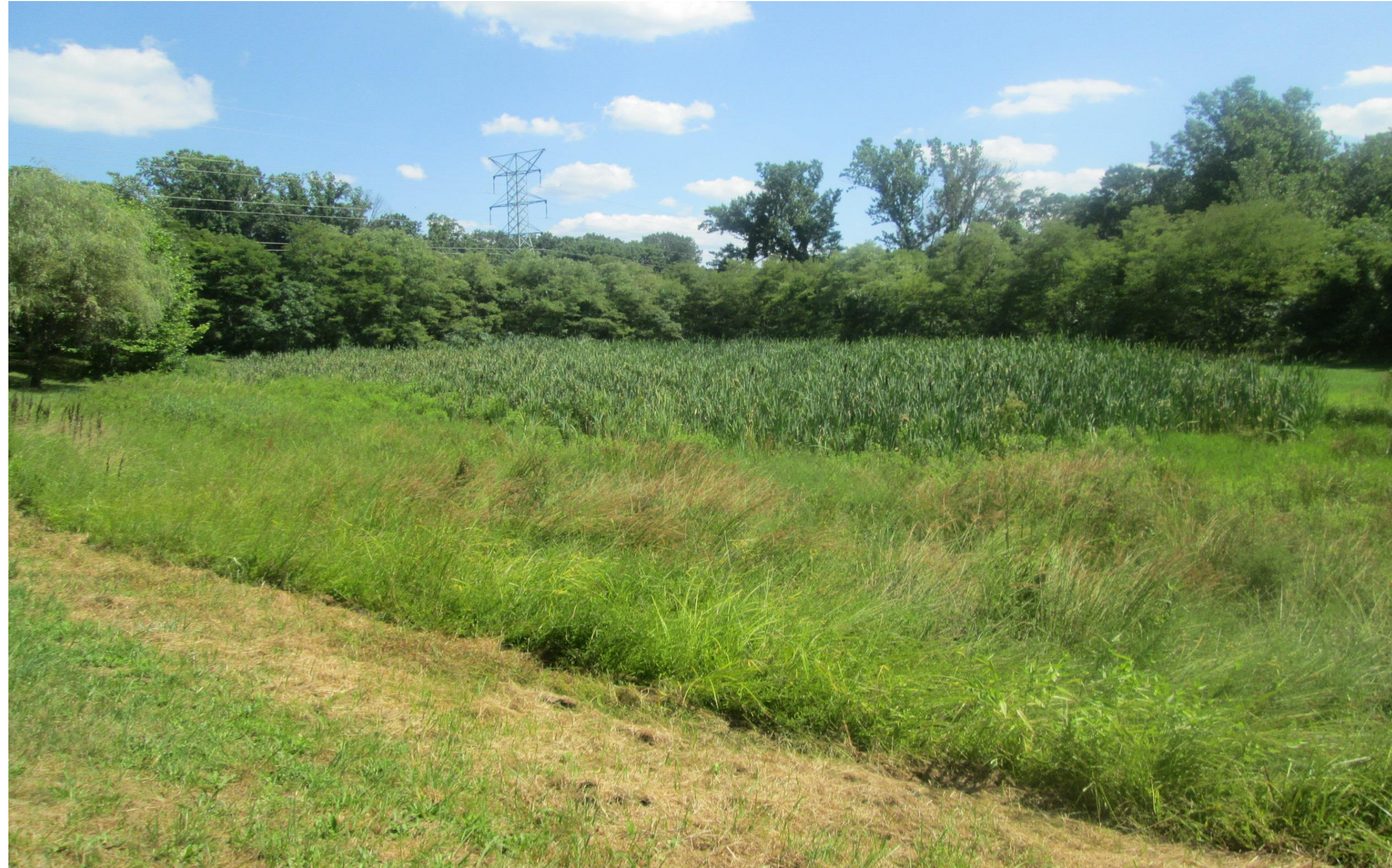
Overview of basin
