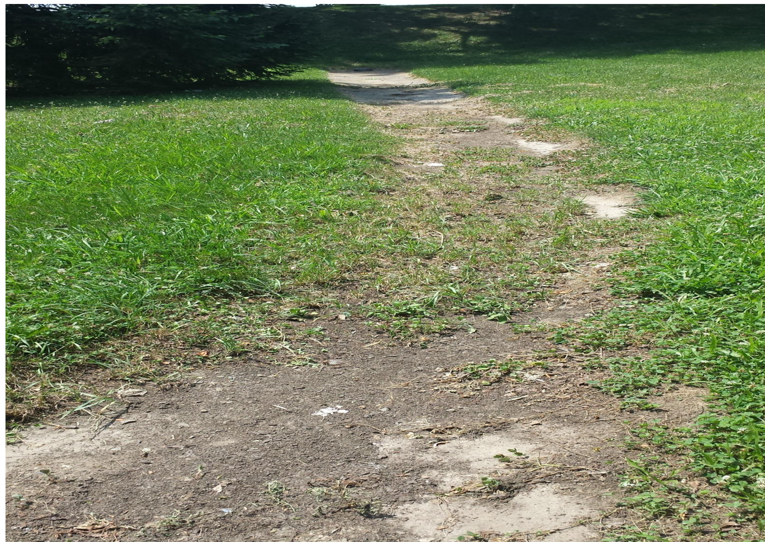
Overgrown on low flow channel
