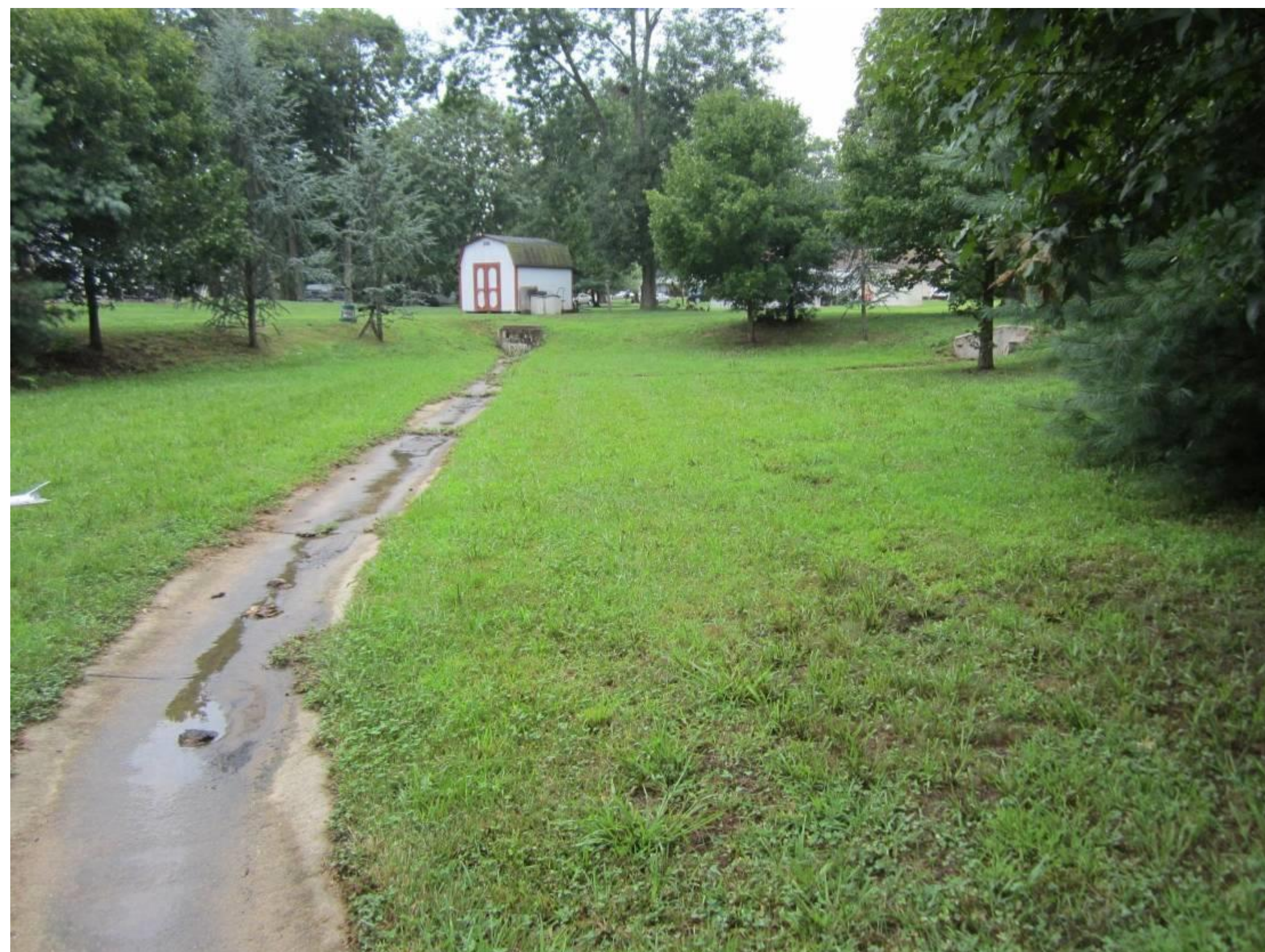
Basin bottom looking southwest
