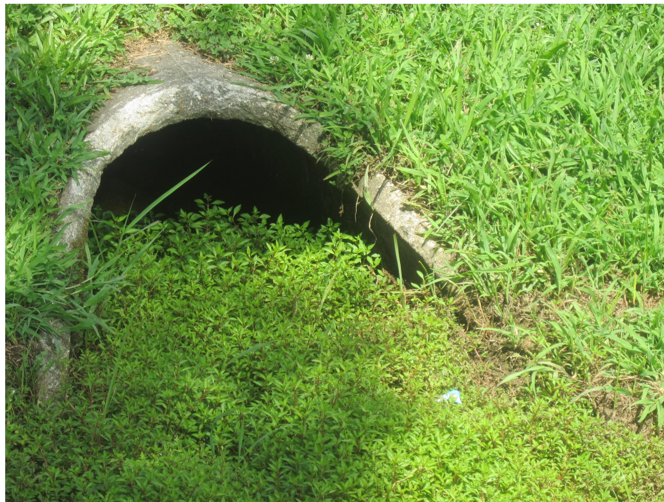
Basin #160 outlet structure
