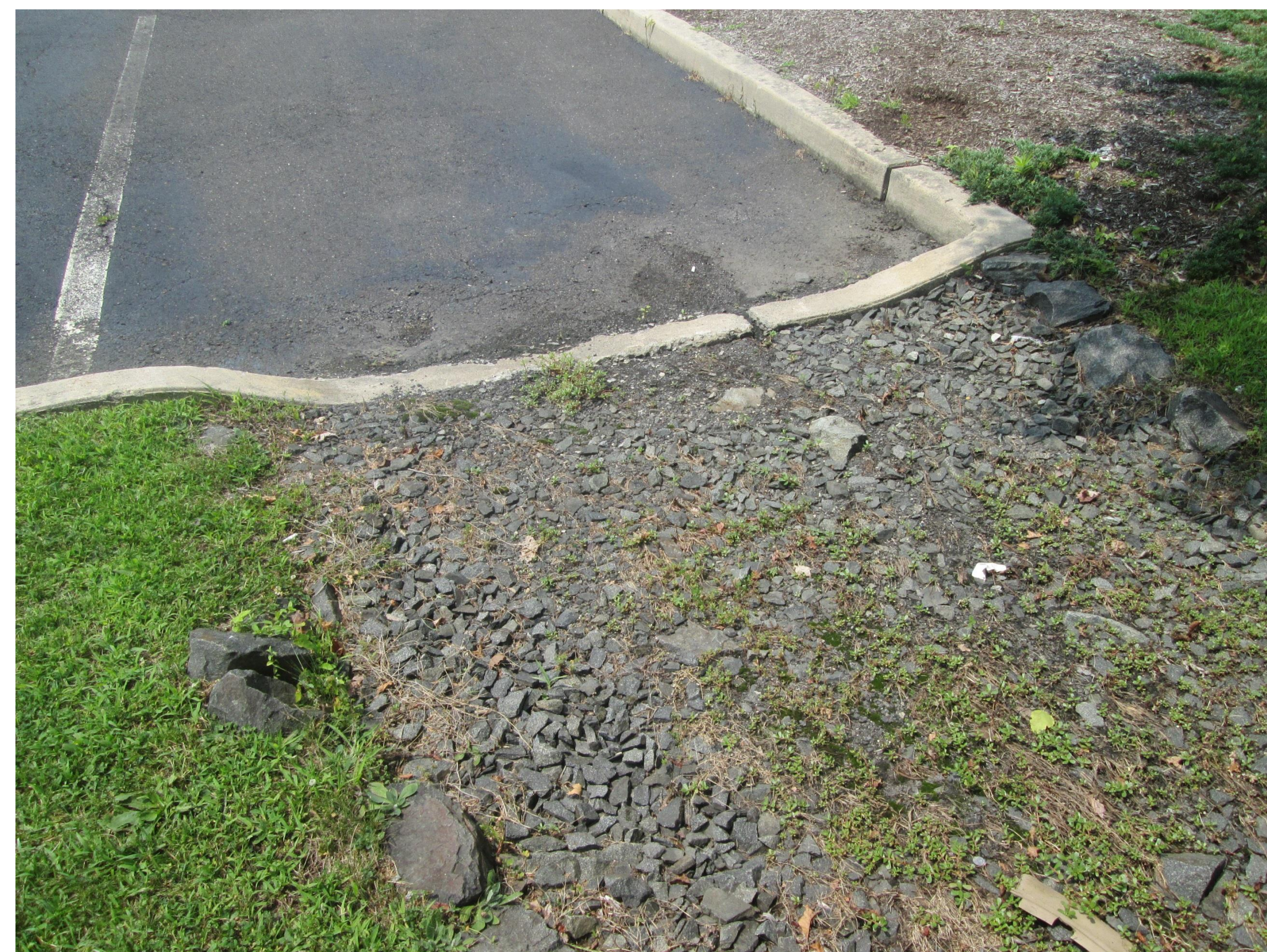
Curb-cut leading to basin
