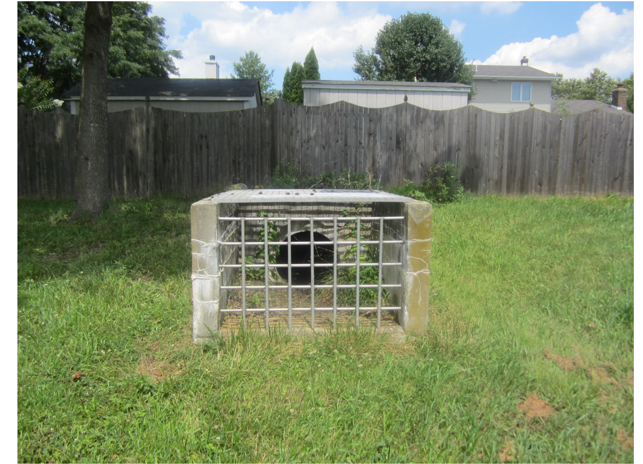
Secondary emergency overflow
