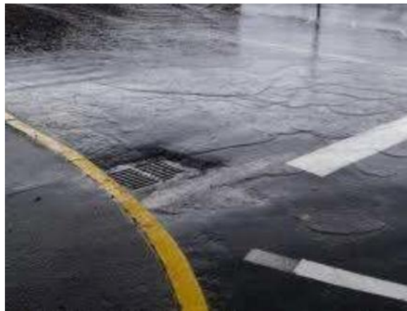
Figure 1: Stormwater draining from a parking lot
