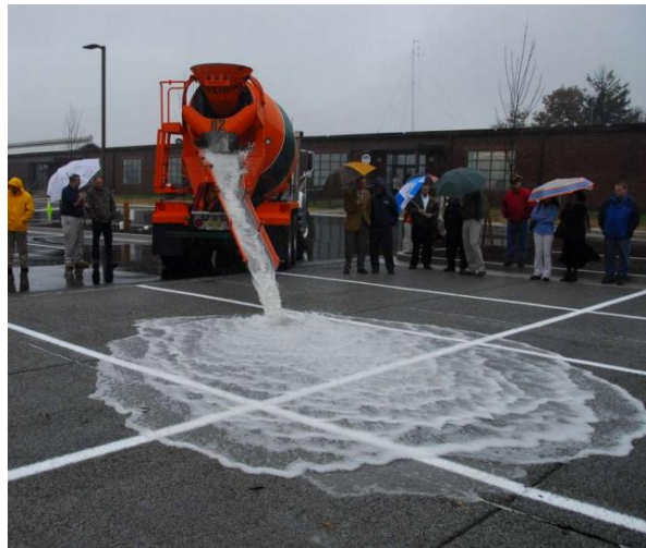
Figure 2: Rapid infiltration of water through porous pavement is demonstrated at the USEPA Edison New Jersey test site
