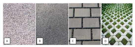
Permeable surfaces: (A) pervious concrete, (B) porous asphalt, (C) interlocking concrete pavers, (D) grid pavers (Rowe, 2012)
