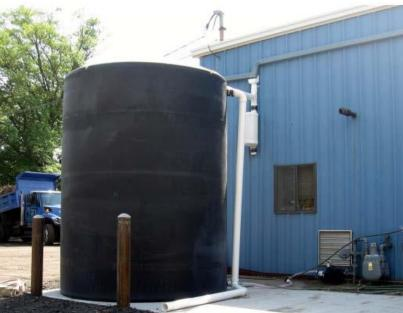
Figure 8b: A 5,000 gallon cistern used to disconnect the rooftop of the Department of Public Works in Clark Township to harvest rainwater for nonprofit car wash events
