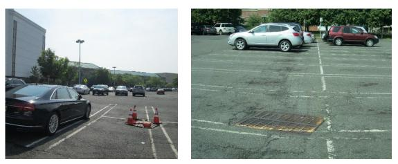
Along the east side of the mall, near the Lord & Taylor department store, pavement is eroded around existing catch basins. Parking spaces can be replaced with pervious pavement collect and infiltrate runoff before it reaches these catch basins. A preliminary soil assessment suggests that more soil testing would be required before determining the soil's suitability for green infrastructure.
