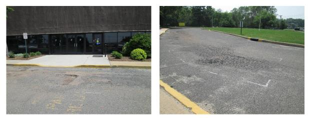
The parking lot is very eroded. Parking spaces can be replaced with pervious pavement to collect and infiltrate runoff. Two rain gardens can also be installed capture, treat, and infiltrate driveway runoff. A preliminary soil assessment suggests that more soil testing would be required before determining the soil's suitability for green infrastructure
