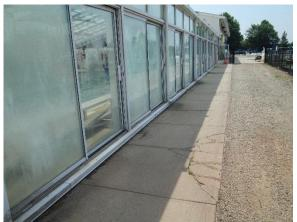
There is a sidewalk along the enclosed pool that is severely eroded, and can be replaced with pervious pavement to allow water to infiltrate. Rain gardens can also be installed to capture, treat, and infiltrate roof runoff. A preliminary soil assessment suggests that the soils have suitable drainage characteristics for green infrastructure.
