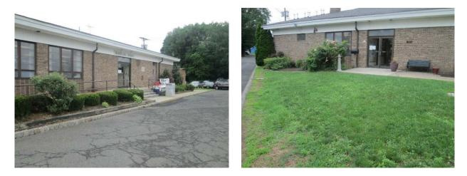
The parking lot runoff can be treated with strategic use of pervious pavement. Half of the roof runoff can be managed with a rain garden on the street side, while the other half can be captured by the pervious pavement. A preliminary soil assessment for this site suggests that soils have suitable drainage characteristics for green infrastructure.
