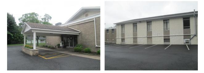
With the exception of the entrance overhang, downspouts currently connect roof runoff directly into the underground sewer system. Downspouts adjacent to the sidewalk can be disconnected into planter boxes, while downspouts by the parking lot can be disconnected into pervious pavement. A preliminary soil assessment for this site suggests that soils have suitable drainage characteristics for green infrastructure.
