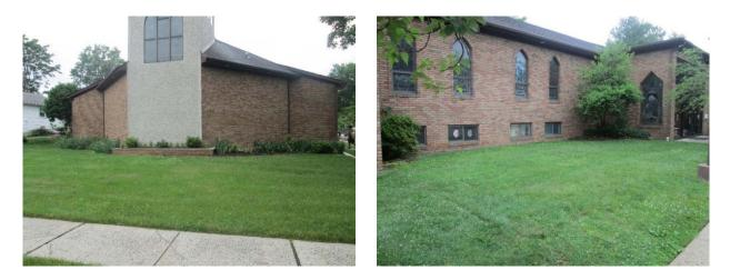
Roof runoff currently flows through both connected and disconnected downspouts. Two rain gardens can be used to capture, treat and infiltrate this runoff. One downspout can also be disconnected into a rain barrel to water the landscaping. A preliminary soil assessment for this site suggests that soils have suitable drainage characteristics for green infrastructure.
