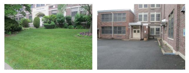
Disconnected downspouts primarily flow directly into street-side storm drains. Porous pavement can be used to capture this runoff. Connected downspouts at the front of the high school can be disconnected into a rain garden. A preliminary soil assessment for this site suggests that soils have suitable drainage characteristics for green infrastructure.
