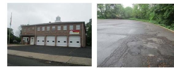
Roof runoff flows into a catch basin at the street and into an adjacent creek. The paved area can be treated with strips of pervious pavement to capture this runoff. Some downspouts can also be routed into a cistern to harvest stormwater and wash the fire trucks. A preliminary soil assessment for this site suggests that soils have suitable drainage characteristics for green infrastructure.
