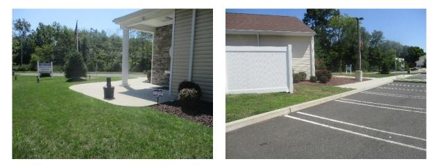
Parking spaces can be replaced with porous asphalt to capture and infiltrate stormwater. The installation of rain gardens adjacent to the building can capture, treat, and infiltrate roof runoff. A preliminary soil assessment suggests that the soils have suitable drainage characteristics for green infrastructure.
