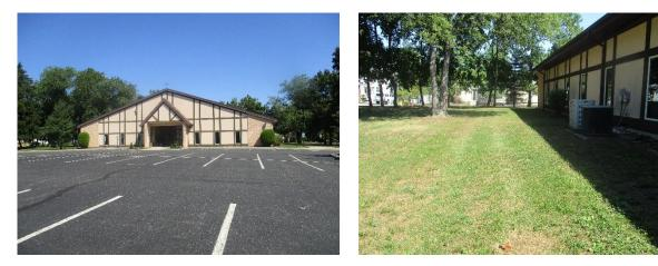
Parking spots can be replaced with porous asphalt to capture and infiltrate stormwater. Rain gardens can capture, treat, and infiltrate roof runoff. A preliminary soil assessment suggests that the soils have suitable drainage characteristics for green infrastructure.
