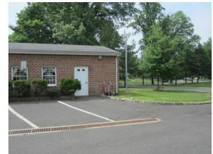
A bioswale and rain gardens can capture, treat and infiltrate parking lot and roof runoff. On the southwest side of the main building, a downspout that drains into a catch basin can also be redirected into a cistern. The harvested rainwater can be used for washing emergency vehicles. A preliminary soil assessment suggests that more soil testing would be required before determining the soil's suitability for green infrastructure.
