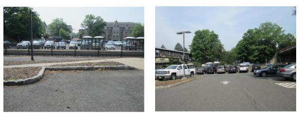
The driveway and parking lot are pitched toward several catch basins draining to local waterways. Parking spaces can be repaved with porous asphalt to promote stormwater infiltration in the parking lots on either side of the train tracks. A preliminary soil assessment suggests that more soil testing would be required before determining the soil's suitability for green infrastructure.
