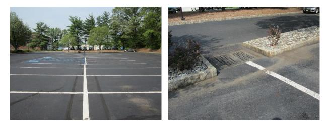
The parking lot is pitched toward the center. Parking spaces in the center of the lot can be repaved with porous asphalt to help manage stormwater. A preliminary soil assessment suggests that more soil testing would be required before determining the soil's suitability for green infrastructure.
