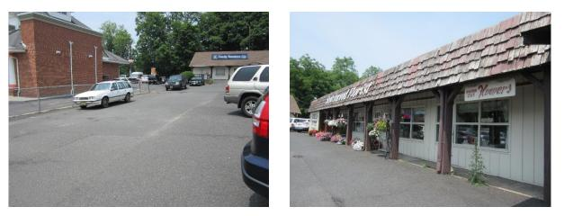
The parking lot is pitched toward the southwest end of the site. The parking spaces at this end can be repaved with porous asphalt to capture stormwater runoff. Roof runoff from the florist shop on the east side of the property can be harvested to water the plants displayed outside the shop by installing a cistern or rain barrel. A preliminary soil assessment suggests that more soil testing would be required before determining the soil's suitability for green infrastructure.
