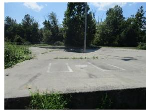
Parking spaces adjacent to the main building can be replaced with pervious pavement to capture and infiltrate stormwater runoff. A preliminary soil assessment suggests that the soils have suitable drainage characteristics for green infrastructure.
