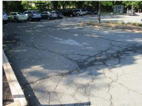
Parking spaces can be replaced with porous asphalt to infiltrate parking lot runoff. A preliminary soil assessment suggests that the soils have suitable drainage characteristics for green infrastructure.
