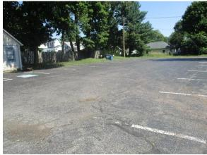
Parking spots can be replaced with pervious pavement to capture and infiltrate runoff. A bioretention system can be installed to capture, treat, and infiltrate roof runoff by disconnecting and redirecting a nearby downspout into it. A preliminary soil assessment suggests that the soils have suitable drainage characteristics for green infrastructure.
