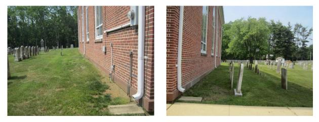
Roof runoff currently flows into six disconnected downspouts. Each downspout can be rerouted into planter boxes to reuse this runoff. A preliminary soil assessment suggests that the soils have suitable drainage characteristics for green infrastructure.
