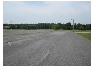
This site has both connected and disconnected downspouts; disconnected downspouts flow onto the grass. The parking lot also flows into the surrounding turf grass. Rain gardens can be installed to capture, treat, and infiltrate this runoff, as well as some roof runoff. A preliminary soil assessment suggests that the soils have suitable drainage characteristics for green infrastructure.
