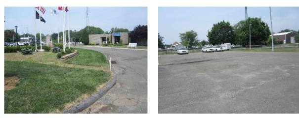
Several buildings have either connected downspouts or internal drainage. One building has disconnected downspouts that releases runoff onto the grass. Bioretention systems can be installed to capture, treat, and infiltrate both roof and parking lot runoff. A preliminary soil assessment suggests that the soils have suitable drainage characteristics for green infrastructure.
