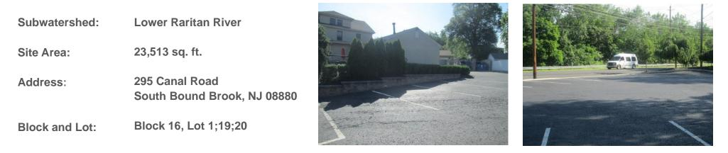
The paved areas are pitched to the street. Parking spaces on the west and northeast sides of the building can be replaced with pervious pavement. The west side can also capture rooftop runoff from existing downspouts. A preliminary soil assessment suggests that the existing soils have suitable drainage characteristics for green infrastructure.
