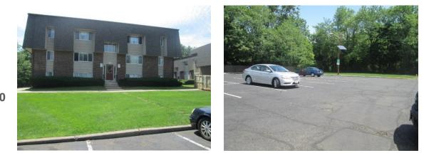
The apartment complex has large areas of pavement for parking that drain to catch basins. Portions of the parking lot can be replaced with porous asphalt to capture and infiltrate stormwater. Bioretention systems can be installed around the apartments to capture and treat roof runoff. A preliminary soil assessment suggests that further testing will need to be done to determine if it has suitable drainage characteristics for green infrastructure.
