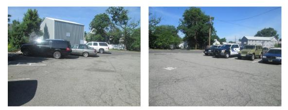
The parking lot slopes toward the building, down the driveway, and into the street. Parking spots can be replaced with porous asphalt to infiltrate stormwater. A preliminary soil assessment suggests that the existing soils have suitable drainage characteristics for green infrastructure.
