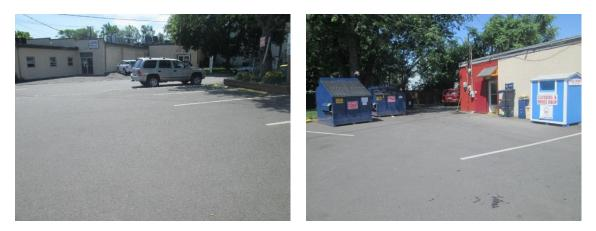
The paved parking lot drains toward the street. Pervious pavement could be utilized in the parking spaces to allow infiltration of runoff before it reaches the street's drainage system. A preliminary soil assessment suggests that the existing soils have suitable drainage characteristics for green infrastructure.
