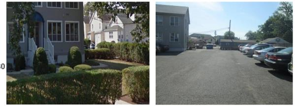
The building's parking lot slopes toward the road. Pervious pavement can be installed in the parking spaces near the building to capture this runoff. In front of the building the turf grass area can be converted into a bioretention system, and downspouts can be disconnected and redirected to allow roof runoff to infiltrate. A preliminary soil assessment suggests that the existing soils have suitable drainage characteristics for green infrastructure.
