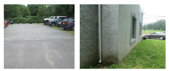
Stormwater from this site flows from the paved parking lot, and from the roof through disconnected downspouts. The downspouts can be redirected to infiltrate into the turf grass, and the parking spaces can be converted into pervious pavement to capture runoff. The gravel area should remain as it is partially pervious. A preliminary soil assessment suggests that more soil testing would be required before determining the soil's suitability for green infrastructure.
