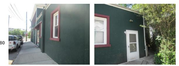
The building's downspouts are directly connected to the sewer system. Downspouts can be disconnected into planter boxes to treat the roof runoff before flowing into the street's drainage system. A preliminary soil assessment suggests that the existing soils have suitable drainage characteristics for green infrastructure.
