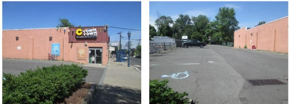
The parking lots drain through a series of catch basins. The building has connected downspouts which can be disconnected, and pervious pavement can be used in the parking lot to capture both road and roof stormwater runoff. A preliminary soil assessment suggests that the existing soils have suitable drainage characteristics for green infrastructure.
