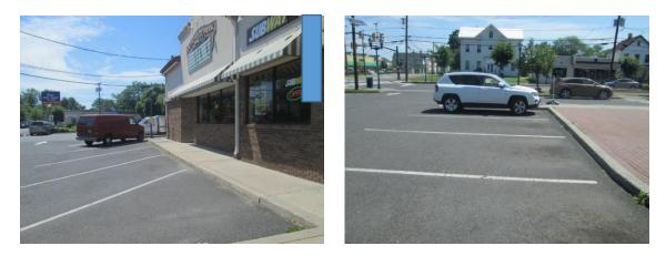
The runoff from the parking area can be captured if the parking spaces were converted to pervious pavement. The building has disconnected downspouts which can be redirected into downspout planter boxes to treat the runoff from the roof. A preliminary soil assessment suggests that the existing soils have suitable drainage characteristics for green infrastructure.
