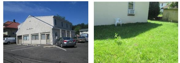
Two downspouts at the rear of the building can be redirected into a rain garden to capture and treat roof runoff. The paved area drains to the street. Pervious pavement can be used in the parking spaces to capture stormwater from the this area and roof runoff from disconnected downspouts next to these spaces. A preliminary soil assessment suggests that more soil testing would be required before determining the soil's suitability for green infrastructure.
