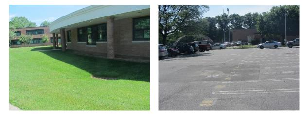
Parking spots can be replaced with pervious pavement to capture and infiltrate stormwater. Rain gardens can be installed to capture, treat, and infiltrate roof runoff. A preliminary soil assessment suggests that more soil testing would be required before determining the soil's suitability for green infrastructure.
