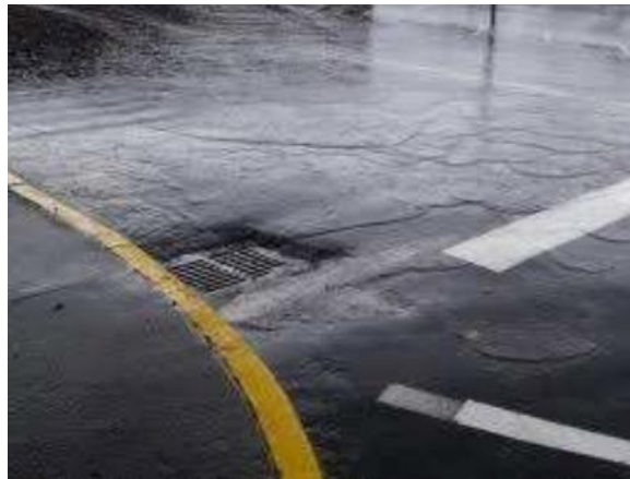
Figure 1: Stormwater draining from a parking lot
