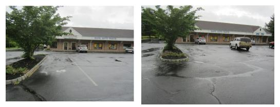
Pervious pavement can be installed in the center spots of the parking lot in front of the site to help collect the runoff from the drainage area and downspouts to prevent further pooling, erosion, and runoff contamination. The rooftop drainage area can also be treated with downspout planter boxes.
