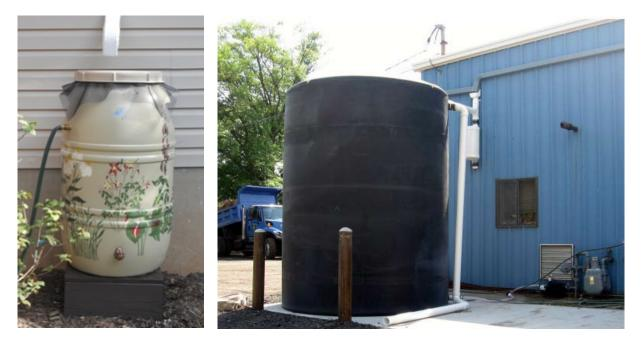
Figure 8a: Rain barrel used to disconnect a downspout with the overflow going to a flower bed
