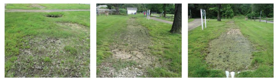
Connected bioretention systems can be installed on the eastern edge of the parking lot to capture, treat, and infiltrate runoff. The systems can be linked by pipes (already installed) shown in the above image. Pervious pavement can be installed in the parking spaces on the southern edge of the parking lot to filter and infiltrate pavement runoff. A preliminary soil assessment suggests that more soil testing would be required before determining the soil's suitability for green infrastructure.
