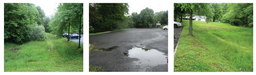
A rain garden can be installed to reduce the flooding that occurs east of the parking lot. Pervious pavement can be installed in the parking lot row directly west of the building to capture stormwater runoff from both the parking lot and the rooftop. A preliminary soil assessment suggests that more soil testing would be required before determining the soil's suitability for green infrastructure.
