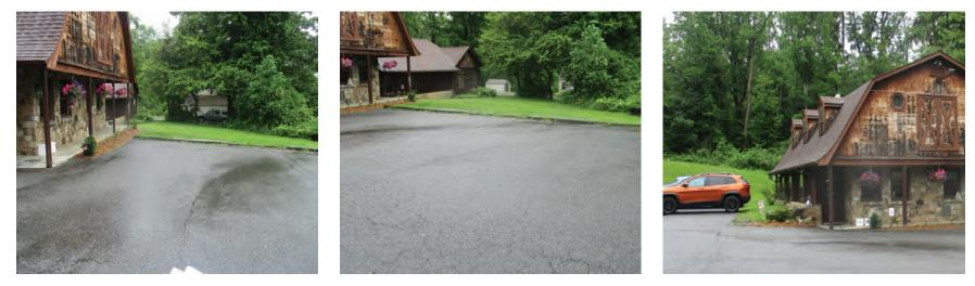
A rain garden can be installed south of the building to capture stormwater runoff from both the rooftop of the building as well as the parking lot. Downspout planter boxes can be installed in front of the building to capture the stormwater runoff from the western rooftop. A preliminary soil assessment suggests that the soils have suitable drainage characteristics for green infrastructure.
