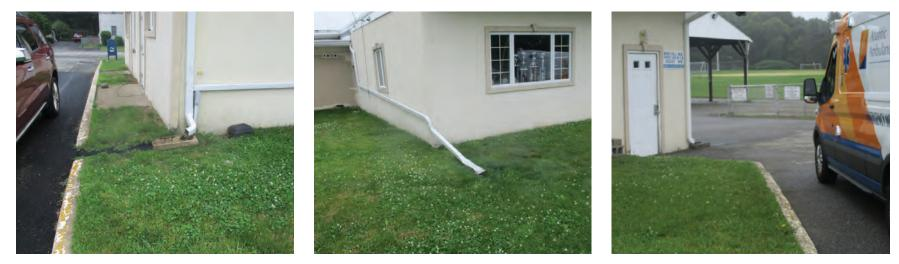
A rain garden can be installed in the turfgrass area near the building to capture, treat, and infiltrate rooftop runoff. A preliminary soil assessment suggests that more soil testing would be required before determining the soil's suitability for green infrastructure.
