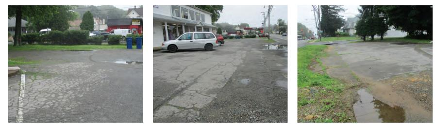
Pervious pavement can be installed on a parking strip south of the building to capture and infiltrate stormwater. A preliminary soil assessment suggests that the soils have suitable drainage characteristics for green infrastructure.
