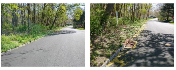
A bioswale can be installed west of the existing catch basin in the grassed area between the tree cover. The catch basin had standing water in it so an investigation to the downhill piping could help with water ponding issues in this area. A preliminary soil assessment suggests that the soils have suitable drainage characteristics for green infrastructure.
