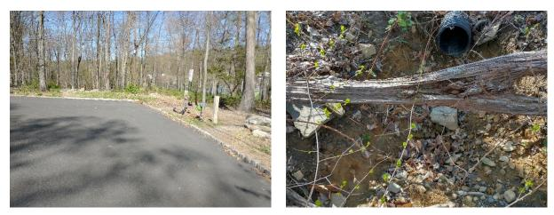
The northwestern section of the pavement can be replaced with a rain garden to intercept stormwater prior to it entering the catch basin. The outfall pipe of the catch basin can be armored with rock to prevent erosion, and the channel downhill of it can be cleared of debris and converted to a bioswale to help promote water infiltration. A preliminary soil assessment suggests that the soils have suitable drainage characteristics for green infrastructure.
