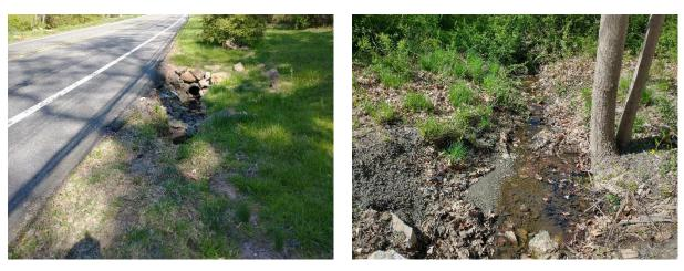
Using an existing curb cut and underground piping system, the daylighted areas can be converted to a bioswale to help promote water infiltration. The outfall pipe on the southern section of the roadway can have the channel cleared of debris, regraded, and planted to be converted to a bioswale. A preliminary soil assessment suggests that the soils have suitable drainage characteristics for green infrastructure.
