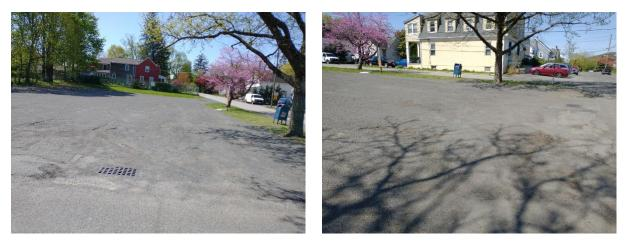
A stormwater planter can be installed uphill of the catch basin to intercept the stormwater prior it entering the basin. A major portion of cost for stormwater planter installation is in the excavation, curbing, and debris removal. The estimated cost is variable and dependent on those factors. A preliminary soil assessment suggests that the soils have suitable drainage characteristics for green infrastructure.
