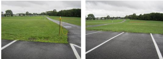
A section of parking spaces can be converted to porous pavement to capture and infiltrate runoff from the parking lot. Overflow runoff can be treated with a rain garden installed in the turfgrass area adjacent to the pervious pavement. A preliminary soil assessment suggests that more soil testing would be required before determining the soil's suitability for green infrastructure.
