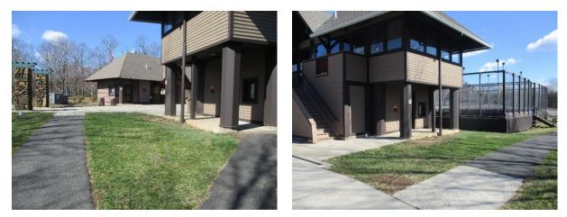
The stormwater runoff coming from the impervious cover in this park center can be captured by a rain garden. A rain garden in this location could provide an eye catching attraction that would improve the overall quality of the park's atmosphere. A preliminary soil assessment suggests that more soil testing would be required before determining the soil's suitability for green infrastructure.
