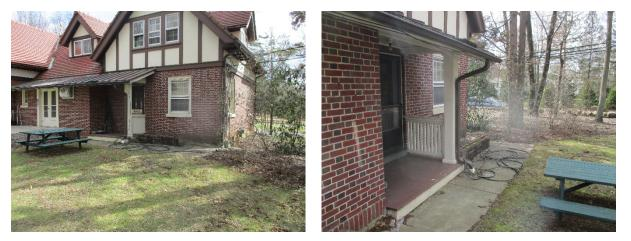
Rain gardens can be installed in the turfgrass area near the entrance of the building and in the rear to capture, treat, and infiltrate stormwater runoff from the parking lot. Downspout planter boxes can be installed to capture and treat stormwater runoff form the rooftop. A preliminary soil assessment suggests that more soil testing would be required before determining the soil's suitability for green infrastructure.
