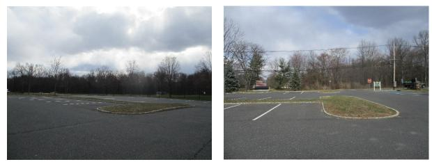
Two sections of parking spaces can be converted to porous pavement to capture and infiltrate stormwater runoff from the parking lot. A preliminary soil assessment suggests that more soil testing would be required before determining the soil's suitability for green infrastructure.
