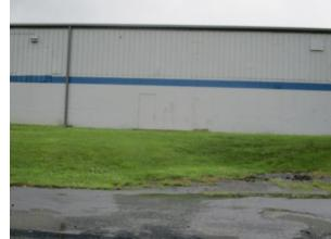
A rain garden can be installed along the front of the building near multiple disconnected downspouts to capture, treat, and infiltrate rooftop runoff. A preliminary soil assessment suggests that more soil testing would be required before determining the soil's suitability for green infrastructure.
