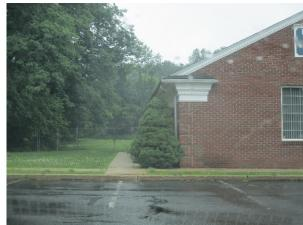
A cistern can be installed on the north side of the public works building near a connected downspout. The water from the cistern can then be used for watering gardens, washing vehicles, or for other non-potable uses. Rain gardens can be installed on the west and east side of the building to capture, treat, and infiltrate rooftop runoff. A preliminary soil assessment suggests that more soil testing would be required before determining the soil's suitability for green infrastructure.
