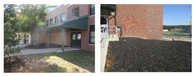
Bioretention systems can be installed near the southeastern entrances in the spaces between the walkways to capture downspout runoff. Pervious pavement can be installed in the northern parking lot to capture and infiltrate the runoff from the parking lot. A preliminary soil assessment suggests that more soil testing would be required before determining the soil's suitability for green infrastructure.
