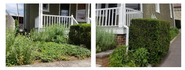
Downspouts on the northwest and southeast corners of the building can be disconnected and converted to planter boxes to capture stormwater runoff from the roof. A preliminary soil assessment suggests that more soil testing would be required before determining the soil's suitability for green infrastructure.
