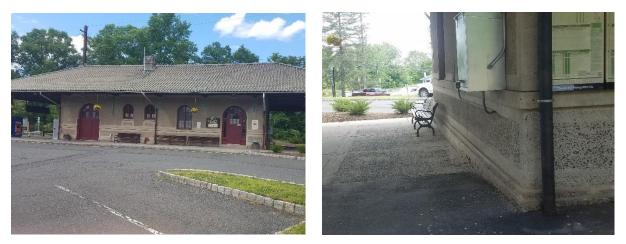
Downspouts on the north and south of the building can be disconnected and converted to planter boxes to capture stormwater runoff from the roof. Sections of parking spaces can be converted to porous pavement to capture and infiltrate stormwater runoff from the parking lot. A preliminary soil assessment suggests that more soil testing would be required before determining the soil's suitability for green infrastructure.
