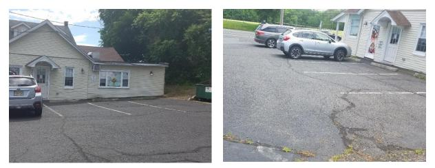
Parking spaces in the parking lot to the north of the building can be converted to porous pavement to capture and infiltrate stormwater runoff from the parking lot and roof. The downspout on the front of the building can be directed to downspout planter boxes to help capture stormwater. A preliminary soil assessment suggests that the soils have suitable drainage characteristics for green infrastructure.
