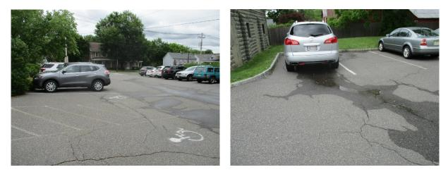
A bioretention system can be installed in the turfgrass area near the brick building to capture, treat, and infiltrate stormwater runoff from the parking lot. The parking spaces east of the entrance can be converted to pervious pavement to help capture additional stormwater runoff. A preliminary soil assessment suggests that more soil testing would be required before determining the soil's suitability for green infrastructure.
