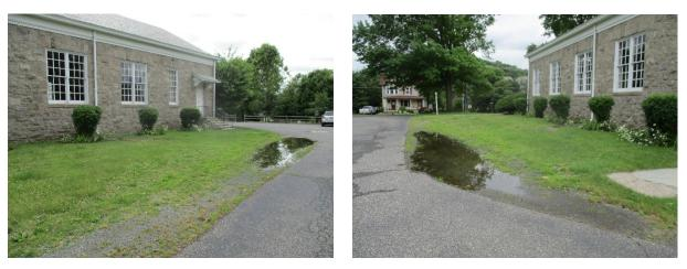
A turfgrass area to the east of the building can be converted to a bioretention system to capture, treat, and infiltrate stormwater runoff from the building's roof. A preliminary soil assessment suggests that more soil testing would be required before determining the soil's suitability for green infrastructure.
