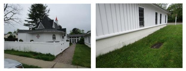
A rain garden can be installed near the rear entrance of the building to capture, treat, and infiltrate the water from five nearby connected downspouts. Two downspout planter boxes can be installed to capture rooftop runoff from different sections of the building. A preliminary soil assessment suggests that the soils have suitable drainage characteristics for green infrastructure.
