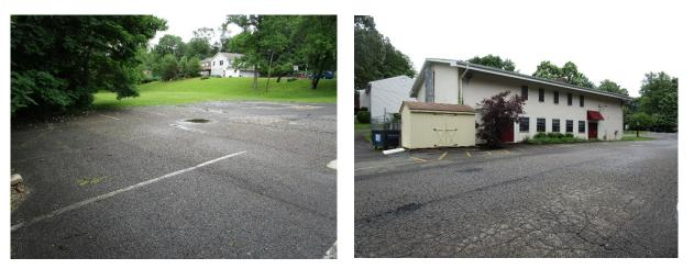
Parking spaces in the parking lot to the northeast of the building can be converted to pervious pavement to capture and infiltrate stormwater runoff from the parking lot. A preliminary soil assessment suggests that more soil testing would be required before determining the soil's suitability for green infrastructure.
