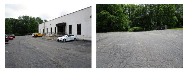
Pervious pavement can be installed in the northeast portion of the parking lot to capture and infiltrate stormwater runoff from the parking area. A preliminary soil assessment suggests that the soils have suitable drainage characteristics for green infrastructure.
