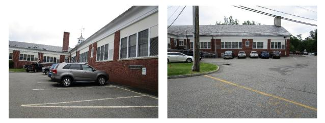
Pervious pavement can be installed in parking spaces throughout the site to capture and infiltrate stormwater runoff from the parking lot and adjacent rooftops. A rain garden can be installed in the area to the south of the building to capture additional stormwater from the rooftop by redirecting downspouts into it. A preliminary soil assessment suggests that the soils have suitable drainage characteristics for green infrastructure.
