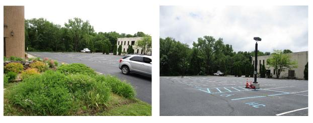
Parking spaces at the southeast end of the parking lot can be converted to pervious pavement to capture and infiltrate stormwater from the parking lot. A preliminary soil assessment suggests that the soils have suitable drainage characteristics for green infrastructure.
