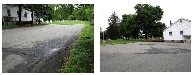
Pervious pavement can be installed south of the building near two disconnected downspouts to capture and infiltrate stormwater runoff from the parking lot and building. Parking spaces in the north parking lot can also be retrofitted with pervious pavement. A preliminary soil assessment suggests that the soils have suitable drainage characteristics for green infrastructure.
