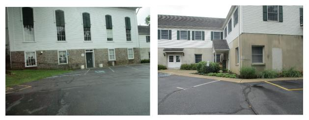
Downspout planter boxes can be constructed at the northeastern downspout. Pervious pavement can be installed along the eastern edge of the parking lot to capture, treat, and infiltrate stormwater runoff from the roof and parking lot. A preliminary soil assessment suggests that more soil testing would be required before determining the soil's suitability for green infrastructure.
