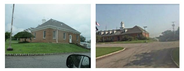
A rain garden can be installed south of the building to capture, treat, and infiltrate stormwater runoff from the roof. Parking spaces in the parking lot to the south can be converted to pervious pavement to capture and infiltrate stormwater runoff from the parking lot. A preliminary soil assessment suggests that more soil testing would be required before determining the soil's suitability for green infrastructure.
