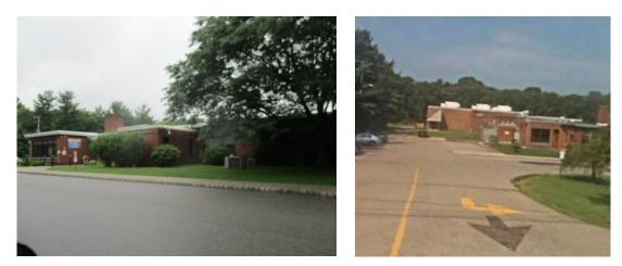
Parking spaces to the south of the school can be converted to pervious pavement to capture and infiltrate stormwater runoff from the street and parking lot. A rain garden can be installed to the east of the building to capture, treat, and infiltrate roof runoff. A preliminary soil assessment suggests that the soils have suitable drainage characteristics for green infrastructure.
