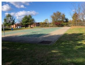
A rain garden can be installed near the playground area to capture, treat, and infiltrate stormwater runoff and also serve as an educational demonstration. Pervious pavement can be installed to treat the drainage area of the basketball court and also improve the structure of the existing cracked pavement. A preliminary soil assessment suggests that the soils have suitable drainage characteristics for green infrastructure.
