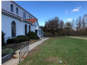
A rain garden can be installed east of the building to capture, treat, and infiltrate runoff from the rooftop. A section of parking spaces can be converted to porous pavement to capture and infiltrate runoff from the parking lot. A preliminary soil assessment suggests that the soils have suitable drainage characteristics for green infrastructure.
