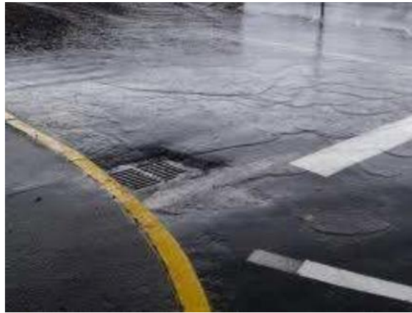
Figure 1: Stormwater draining from a parking lot
