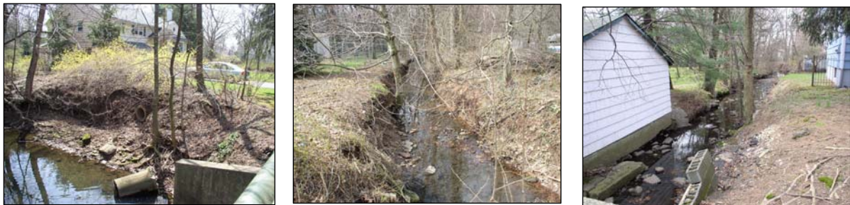
Figure 2: Highly Erodible Soils (left to right)
