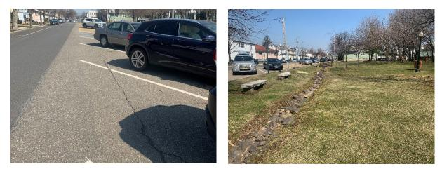
An existing rock swale can be converted to a bioswale to aid in infiltration of the stormwater runoff entering it. Additionally, the parking spaces to the west of the park can be converted to pervious pavement to capture, treat, and infiltrate the stormwater runoff from the parking lot. A preliminary soil assessment suggests that more soil testing would be required before determining the soil's suitability for green infrastructure.
