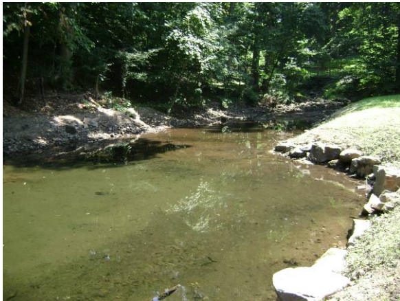
Figure 17a: Poor bank stability in CB1. (Photo: RCE Water Resources Program)
