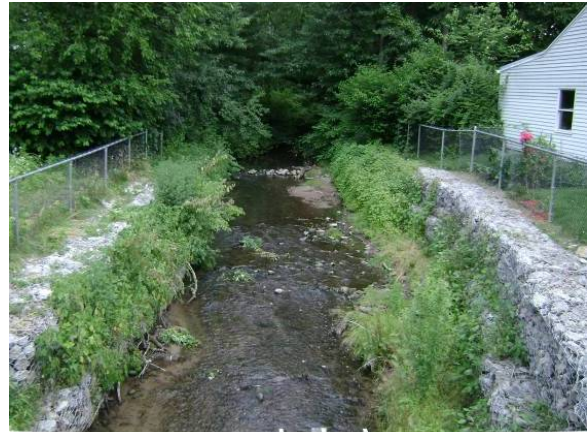
Figure 17b: Example of channelized stream with no pools in CB1. (Photo: RCE Water Resources Program)
