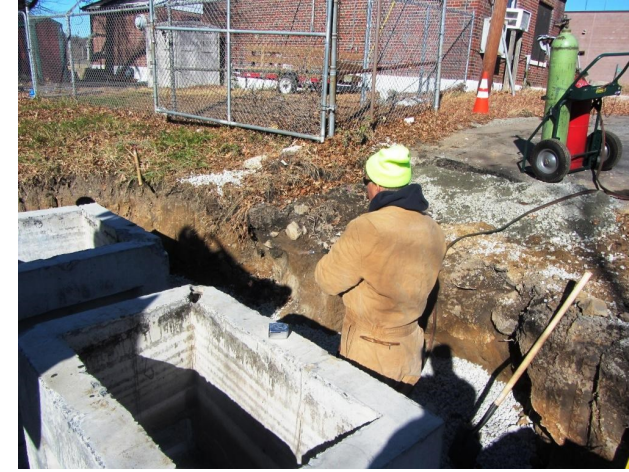
Installation of the sedimentation chamber boxes by Parsippany-Troy Hills DPW staff. Photo credit Pat Rector
