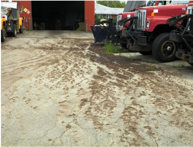
Sediment loading at DPW facilities is often very high. This photograph illustrates sediment at one DPW maintenance yard Photo credit Pat Rector
