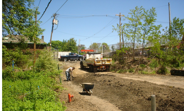
The berm is the low earthen wall of the swale that is planted with upland plants. The berm defines the edge of the swale and helps maintain the flow of the runoff within the channel of the swale.
