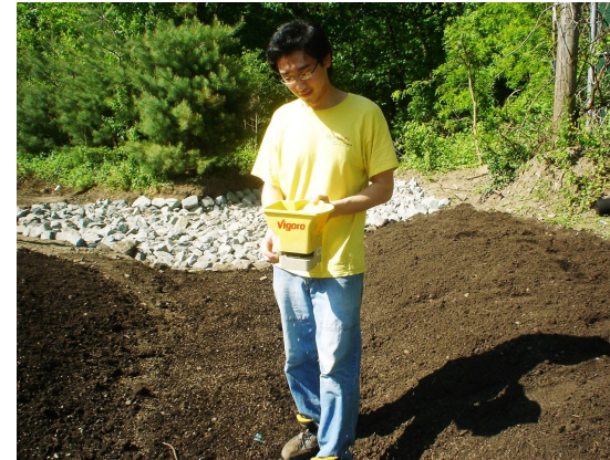
Rutgers student spreading rye grass seed in the channel of the vegetated swale. Photo credit Pat Rector
