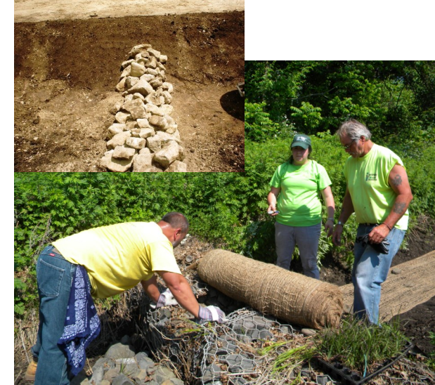
Several check dams were installed in the vegetated swale using rocks in wire cages (also known as gabions). These check dams create a barrier to reduce channel velocity and promote settling of sediments.
