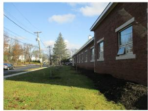
Rain gardens can be installed at each end of the building to capture stormwater runoff from the rooftop. A cistern can be installed in the back to capture and reuse rooftop runoff for non-potable purposes, such as washing vehicles. A preliminary soil assessment suggests that more soil testing would be required before determining the soil's suitability for green infrastructure.
