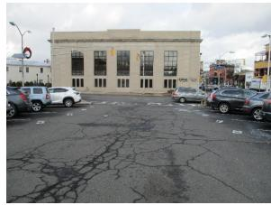
Downspout planter boxes can be installed at the station building to capture and store stormwater runoff from the roof. Additionally, lot #2 can be outfitted with pervious pavement to aid in the infiltration and capture of stormwater runoff. Tree filter boxes can be installed in the islands of lot #8 to capture runoff from the lot. A preliminary soil assessment suggests that more soil testing would be required before determining the soil's suitability for green infrastructure.
