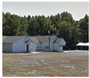
Southwestern parking spaces can be replaced with pervious pavement to capture and infiltrate stormwater from the street, from parts of the roof, and from the rest of the parking lot. Southeastern parking spaces can be replaced by pervious asphalt to infiltrate rooftop runoff from the remainder of the roof and parking lot. A preliminary soil assessment suggests that more soil testing would be required before determining the soil's suitability for green infrastructure.
