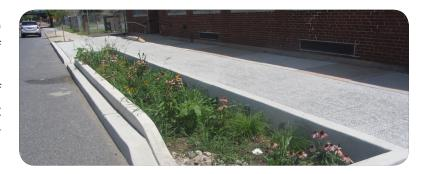
Reduce or convert impervious surfaces. There may be surfaces that are required to be hardened, such as roadways or parking lots, but could be made smaller and still be functional. A parking lot that has two-way cart ways could be converted to one-way cart ways. There also are permeable paving materials such as porous asphalt, pervious concrete, or permeable paving stones that could be substituted for impermeable paving materials.
