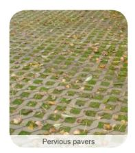
To protect and repair our waterways, reduce flooding, and stop erosion, stormwater runoff has to be better managed. Impervious surfaces need to be disconnected with green infrastructure to prevent stormwater runoff from flowing directly into New Jersey's waterways. Disconnection redirects runoff from paving and rooftops to pervious areas in the landscape.
