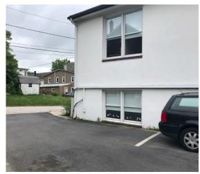
A rain garden can be installed by directing downspouts from the adjacent building into a turfgrass area. The garden will capture, treat, and infiltrate stormwater from the building's rooftop. A preliminary soil assessment suggests that more soil testing would be required before determining the soil's suitability for green infrastructure.
