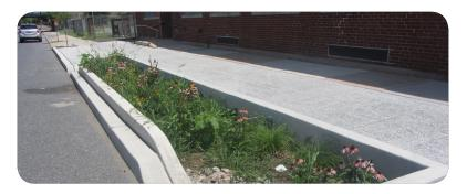
Reduce or convert impervious surfaces. There may be surfaces that are required to be hardened, such as roadways or parking lots, but could be made smaller and still be functional. A parking lot that has two-way cart ways could be converted to one-way cart ways. There also are permeable paving materials such as porous asphalt, pervious concrete, or permeable paving stones that could be substituted for impermeable paving materials.
