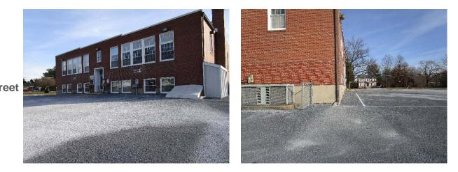
A stormwater planter can be installed along the west side of the municipal building to intercept and infiltrate roof runoff and to provide an aesthetically pleasing addition to the property. Pervious asphalt can replace the parking spaces alongside the northern and southern sides of the lot to capture and infiltrate runoff from the surrounding pavement. A preliminary soil assessment suggests that the soils have suitable drainage characteristics for green infrastructure.
