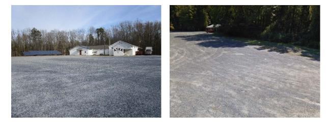
Southwestern parking spaces can be replaced with pervious pavement to capture and infiltrate stormwater from the street, from parts of the roof, and from the rest of the parking lot. Southeastern parking spaces can be replaced by pervious asphalt to infiltrate rooftop runoff from the remainder of the roof and parking lot. A preliminary soil assessment suggests that more soil testing would be required before determining the soil's suitability for green infrastructure.
