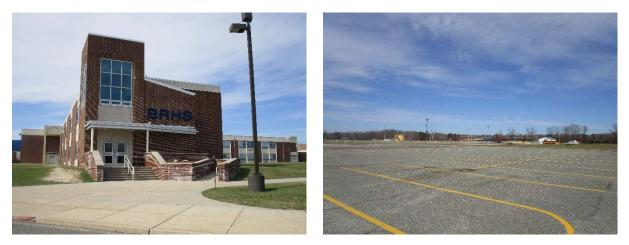
A rain garden can be installed at the corner of one section of parking lot to capture, treat, and infiltrate the associated stormwater runoff. The most southern row of parking spaces can be replaced with pervious pavement to capture and infiltrate stormwater. A preliminary soil assessment suggests that the soils have suitable drainage characteristics for green infrastructure.
