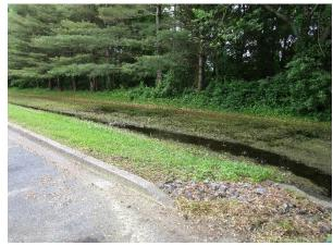
A strip of pervious pavement can be installed along the southeast side of the building where a large volume of stormwater runoff from the site is directed. A preliminary soil assessment suggests that more soil testing would be required before determining the soil's suitability for green infrastructure.
