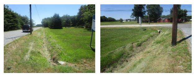
The trench alongside the south side of the road next to the "Canton Baptist Church" sign can be transformed into a rain garden to allow stormwater runoff from the road to infiltrate and reduce contaminant levels more efficiently while providing a habitat for wildlife. A preliminary soil assessment suggests that more soil testing would be required before determining the soil's suitability for green infrastructure.
