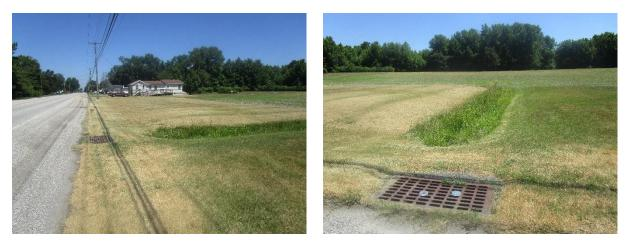
On the east side of the road there exists a bioswale filled with grasses. This can be extended perpendicularly to its current position to create a rain garden, travelling alongside the road to allow stormwater runoff to infiltrate into the ground and reduce contaminant levels. A preliminary soil assessment suggests that more soil testing would be required before determining the soil's suitability for green infrastructure.
