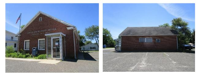
Pervious pavement can be installed in the parking lot to collect stormwater from the three downspouts from the eastern side of the building. A preliminary soil assessment suggests that more soil testing would be required before determining the soil's suitability for green infrastructure.
