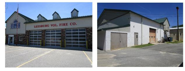
Pervious pavement can be installed on the northeast side of the parking lot to capture and infiltrate the stormwater runoff from the roof. On the south side of the building a connected downspout can be connected to a cistern to capture roof runoff for use in washing cars, watering plants, or for other non-potable purposes. A preliminary soil assessment suggests that more soil testing would be required before determining the soil's suitability for green infrastructure.
