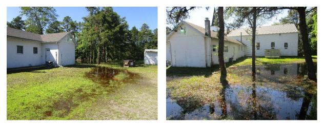
A rain garden can be installed in the front of the building to capture, treat, and infiltrate rooftop runoff. A cistern can be installed along the building to reduce flooding by capturing rooftop runoff, which can later be reused for washing cars or watering gardens. A preliminary soil assessment suggests that more soil testing would be required before determining the soil's suitability for green infrastructure.
