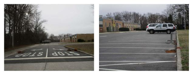
The two parking lots on both the east and west sides of the school can be converted to porous pavement to treat the stormwater runoff from the roof of the elementary school. A preliminary soil assessment suggests that more soil testing would be required before determining the soil's suitability for green infrastructure.
