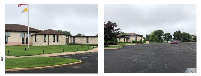
Rain gardens can be installed at several locations around the building to capture, treat, and infiltrate stormwater from the roof. The parking spaces adjacent to the building on the southeast side can be replaced with pervious pavement to capture stormwater from adjacent rooftops and sidewalks. A preliminary soil assessment suggests that the soils have suitable drainage characteristics for green infrastructure.
