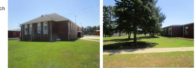
Rain gardens can be installed in the turfgrass areas along the front of the school. The rain gardens will be able to capture and treat runoff from the roof of the school building by directing the downspouts into them. Two downspout planters can be placed along the driveway of the school to help capture runoff from the roof from the downspouts as well. A preliminary soil assessment suggests that the soils have suitable drainage characteristics for green infrastructure.
